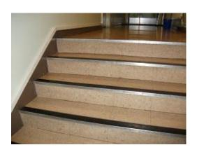
PVC floor tiles & coverings and resin composites, such as bakelite, can contain asbestos. These are typically found in old toilet cisterns and toilet seats; window sills and stair nosings; partitioning; and electrical switchboards, socket outlets and electrical fittings.
