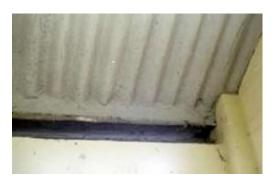
Used mainly for fire protection and insulation, they consist of a high percentage of asbestos usually mixed with a cement binder, applied to beams, columns, ceilings and the underside of floors and canopies. They typically provided fire protection to steelwork and concrete structures in more industrial type buildings and in steel frame buildings. Asbestos fibres can be easily released from sprayed coatings.
