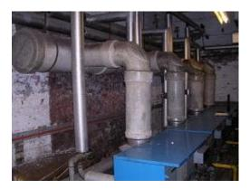
Asbestos insulation products were commonly used in boilers, and on hot water and heating pipe work, for example, asbestos insulation for boilers and pipework in boiler-rooms, underground ducts, and service risers within buildings.
