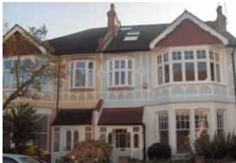
Wooden panel details on Kenilworth Avenue
