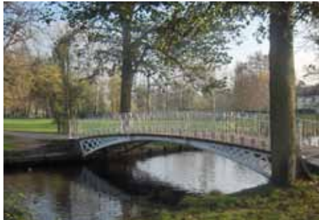
Footbridge over River Wandle
