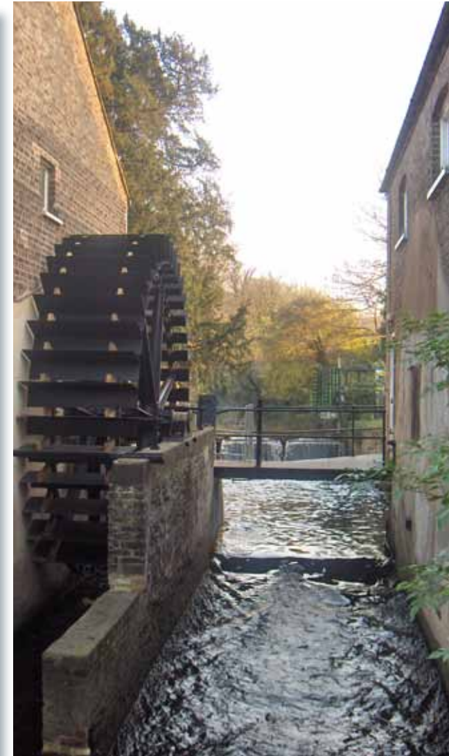
Former snuff mill
