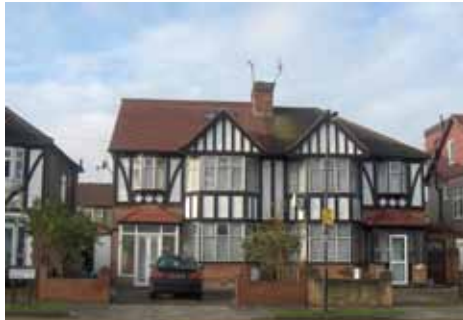
Mock beams Camrose Close
