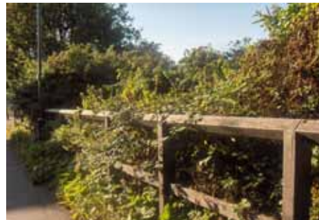
Park perimeter fence
