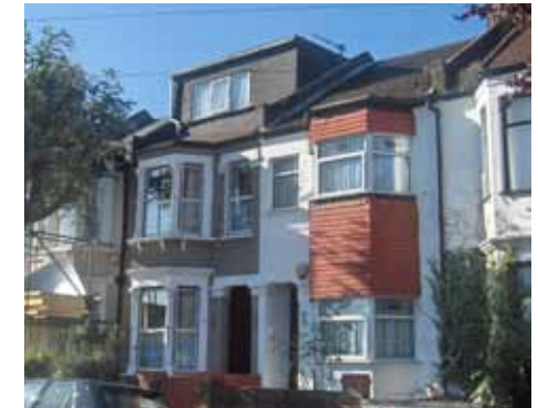
Garfield Road: Oversized front dormer destroys the lines of the original roofs
