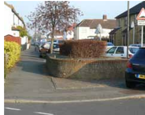
Acacia Road: Planter in need of upgrading
