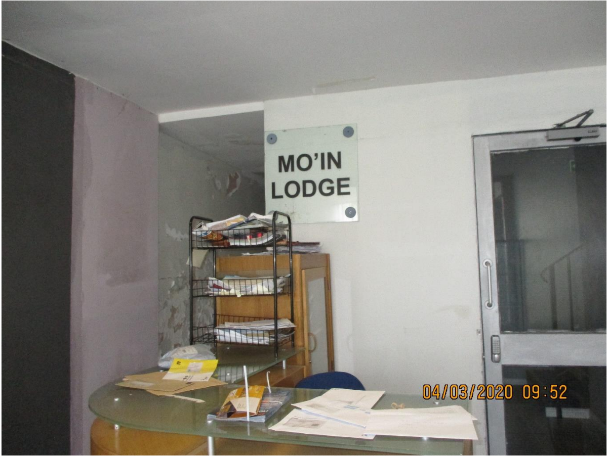
Figure 4 reception area with unsecured post.
