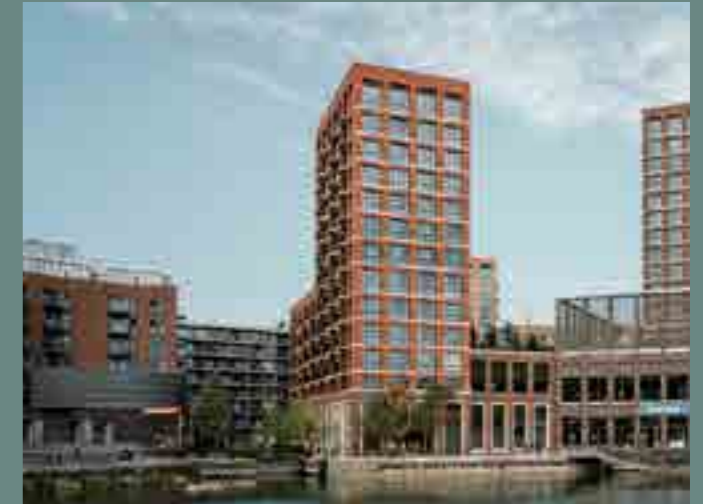
Porters Edge, Southwark © Maccreanor Lavington
