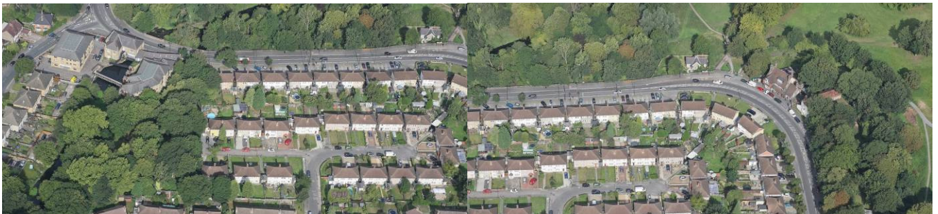
Images above: Southwest & Northwest corners of Ravensbury Village
