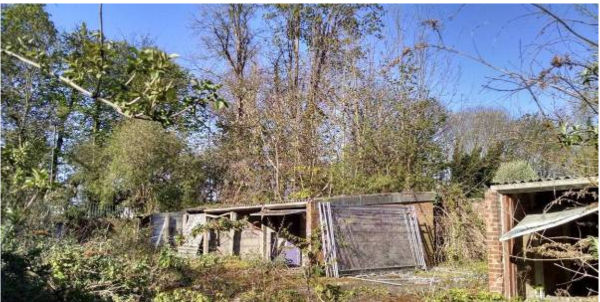
Extent of vegetation within derelict garages site.
