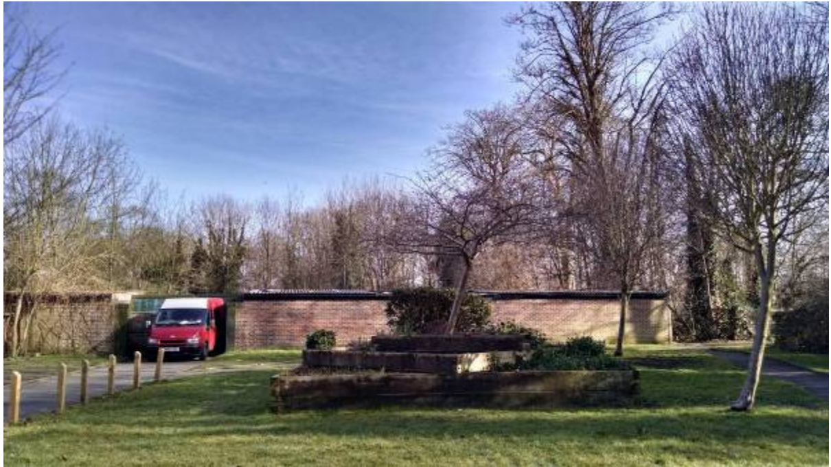
View across existing landscaping towards garages (March 2016)
