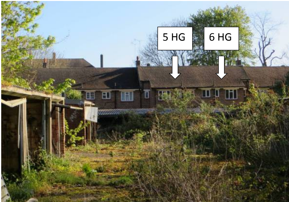
View from within the currently derelict garages site, looking towards Hengelo Gardens with the roof to the 4 storey section of Ravensbury Court visible beyond. Height difference between the derelict garages area & the houses on Hengelo Gardens beyond can be appreciated here.
