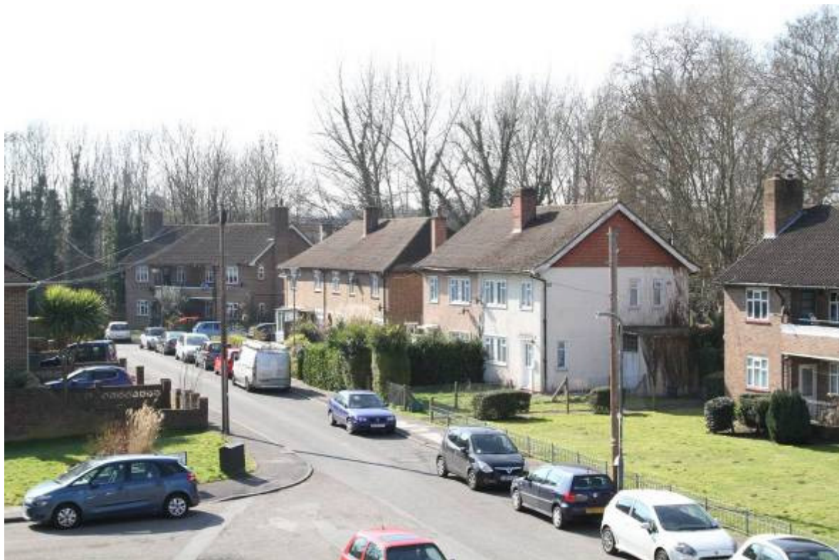
View of Ravensbury Grove from Ravensbury Court, showing two storey heights. Four storeys will represent overdevelopment and will tower over both the park and the existing homes. This will represent an unsustainable form of development in consideration of the conservation status of Ravensbury Park & the Wandle Valley.
