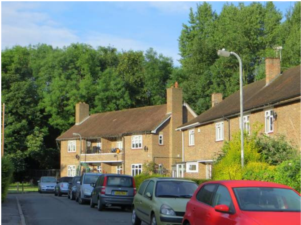
64-70 Ravensbury Grove showing relationship with tree line of Ravensbury Park
