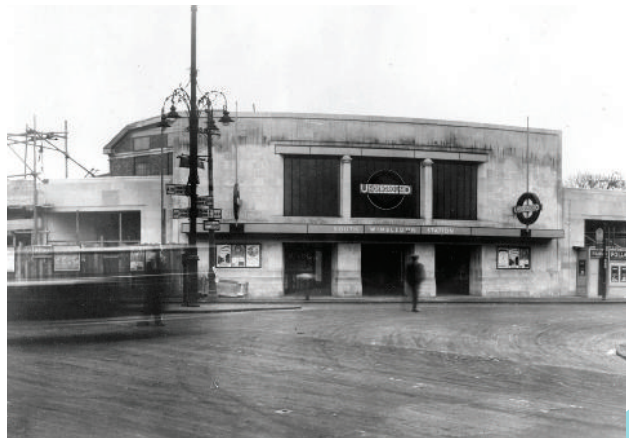
South Wimbledon station 1926
