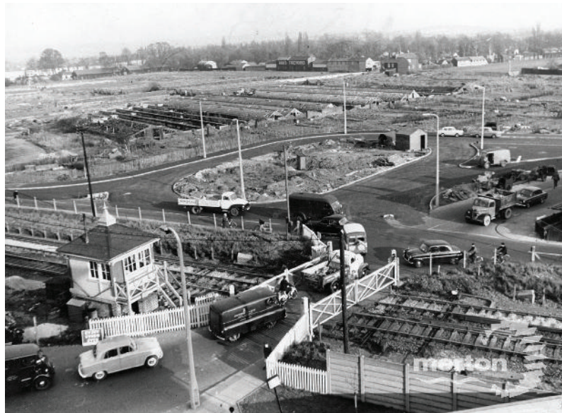
Eastfields level crossing 1961
