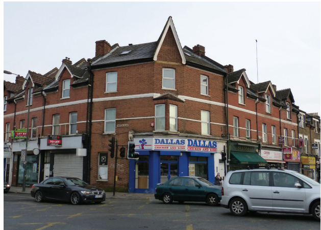
Merton High Street - Merton Road junction
