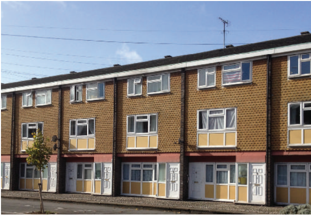
Lack of defensible space
