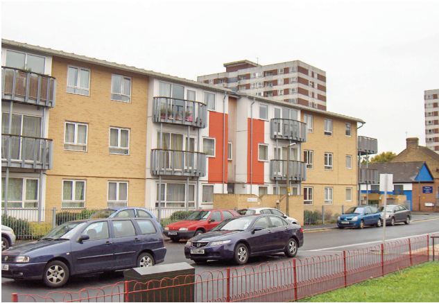
3 storey flats on Nelson Grove Road
