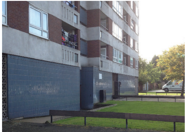
Unclear communal entrance with blank street frontage
