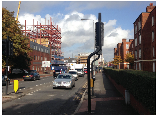
Morden Road (showing Spur House under construction)
