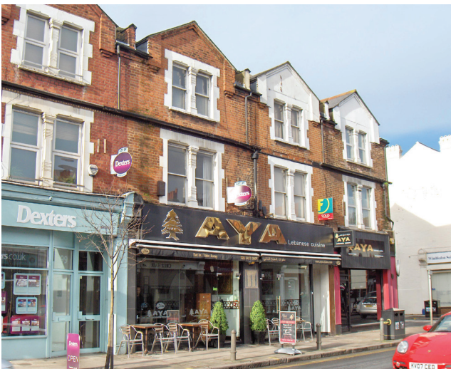
3 storey commercial buildings fronting Merton Road
