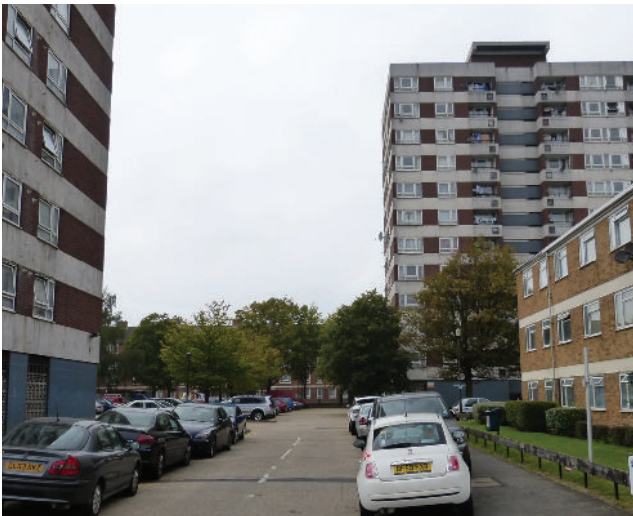
Rear of building block along street frontage
