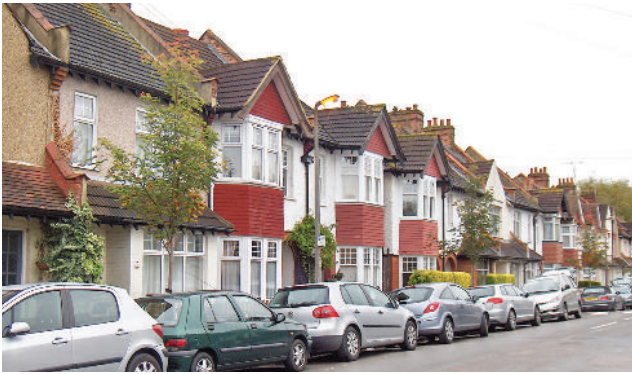
Character area 2: Mill Road
