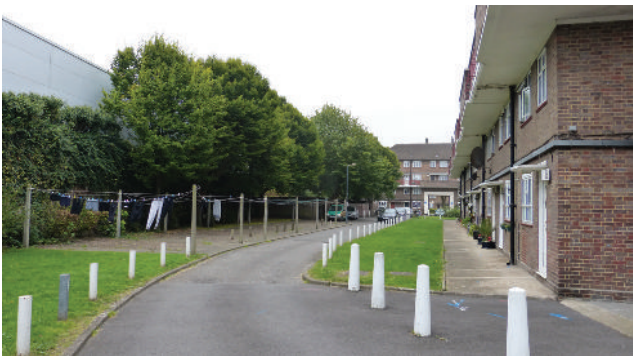
Rear entrances Ravensbury Grove
