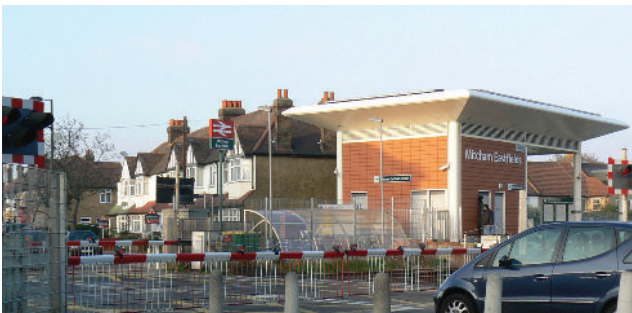
Level crossing at Mitcham Eastfields station
