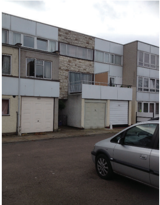
Garage doors dominate ground floor frontages
