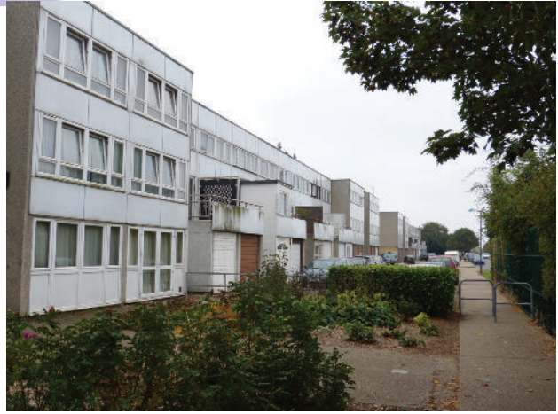
Road closure between Acacia Road and Mulholland Close
