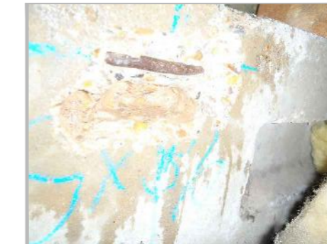
PC3a: VIEW OF B/O C2 TO SECONDARY BEAM
