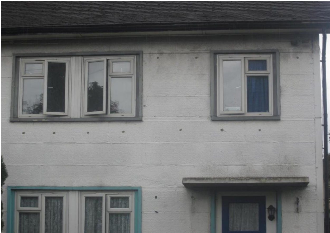
Photograph C18 – Circular markings on elevation
