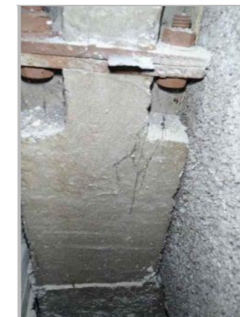
PA11b: VIEW OF COLUMN CONNECTION AT 1ST FLOOR LEVEL
