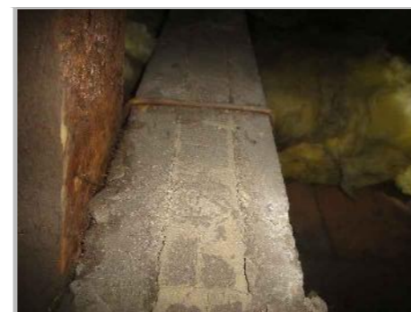
PB2a: VIEW OF INSITU MORTAR PRIOR TO BREAKOUT B/O B1
