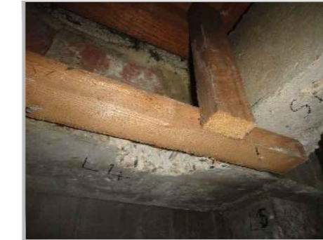
PB6a: GENERAL VIEW OF B/O B7 TO 1ST FLOOR PRIMARY BEAM
