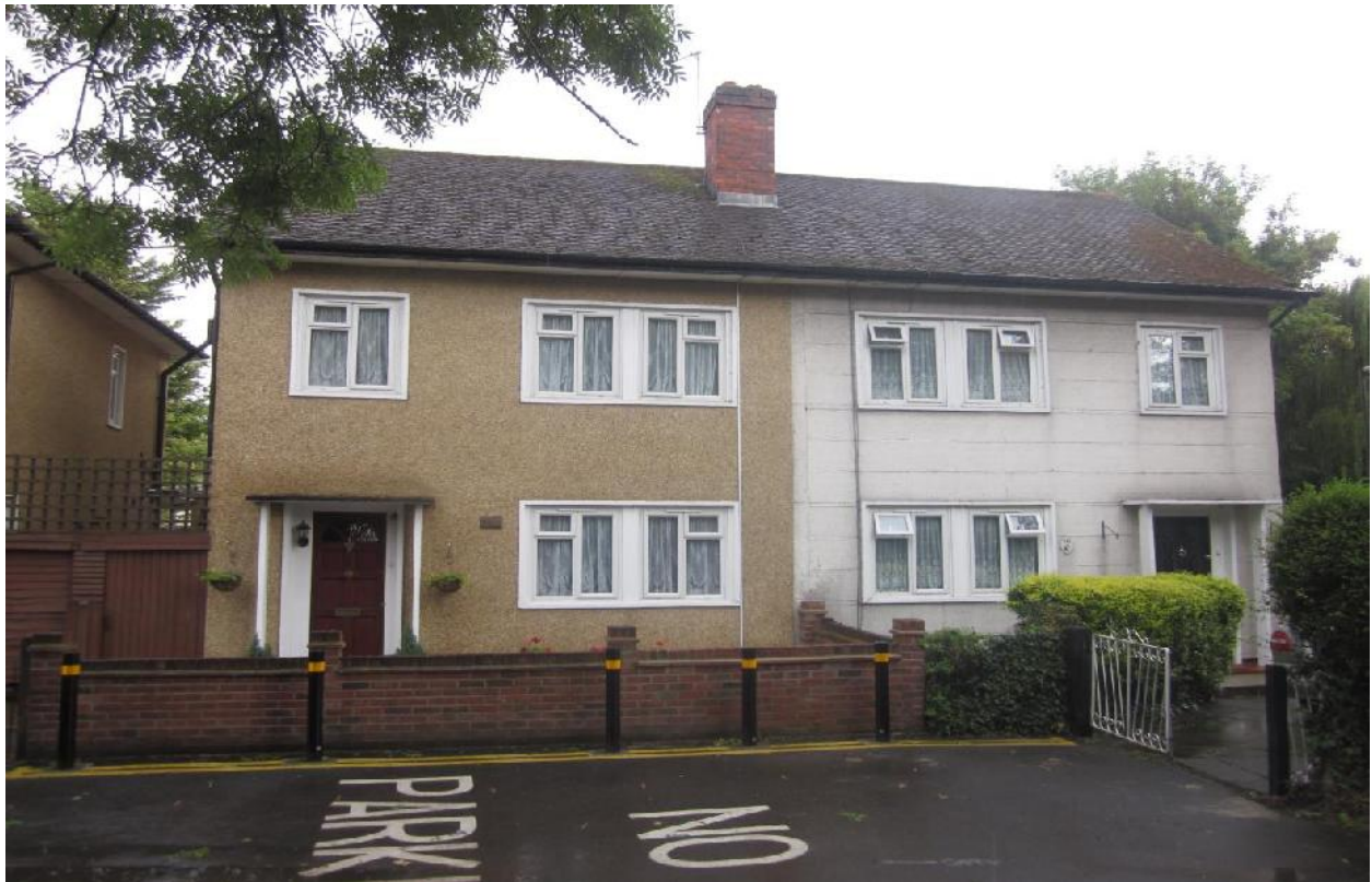
Photograph C20 – Pebble dashed elevation
