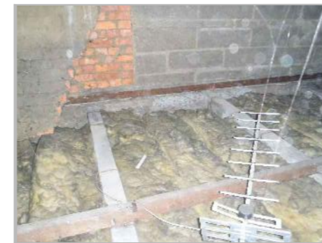
PA2a: VIEW OF SECONDARY BEAMS SPANNING ONTO NORTHERN PRIMARY BEAM
