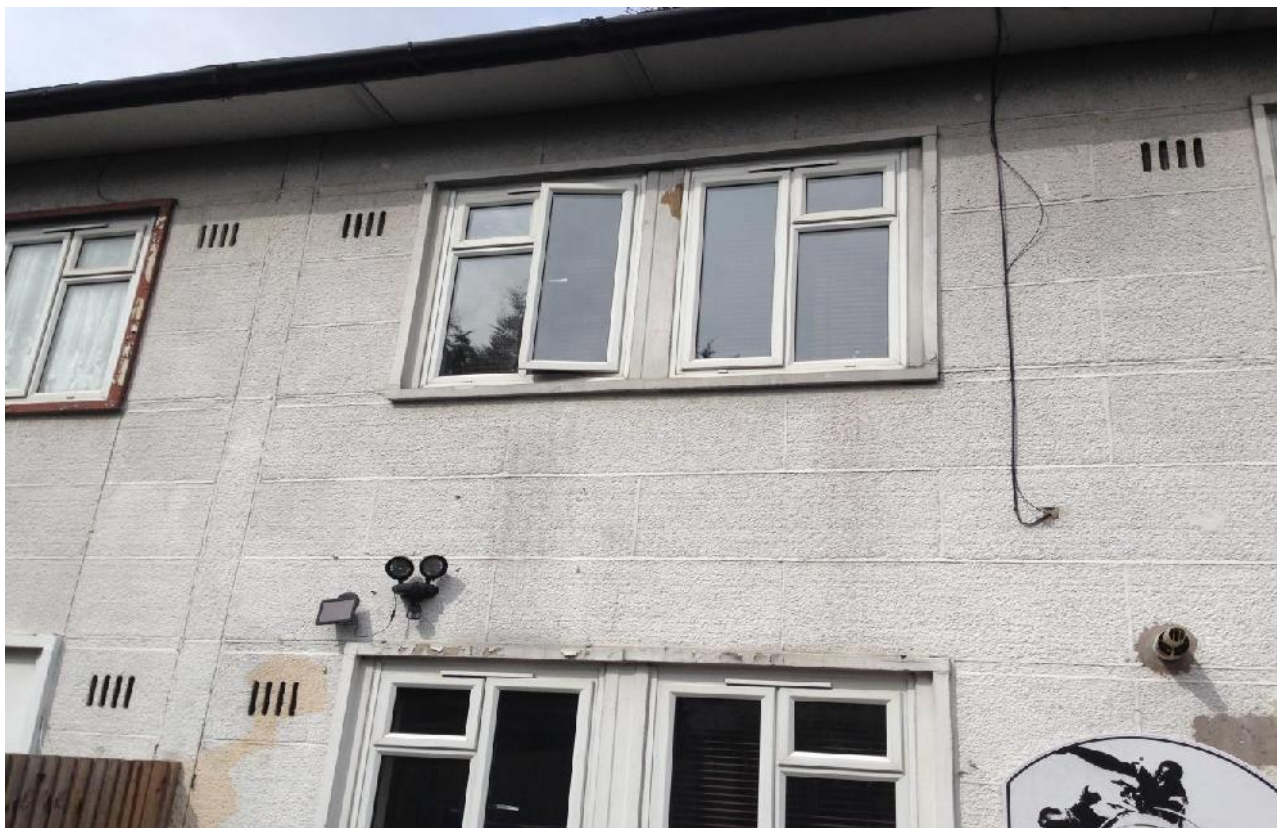
Photograph C8 - 'Grilled' cladding panels in elevation
