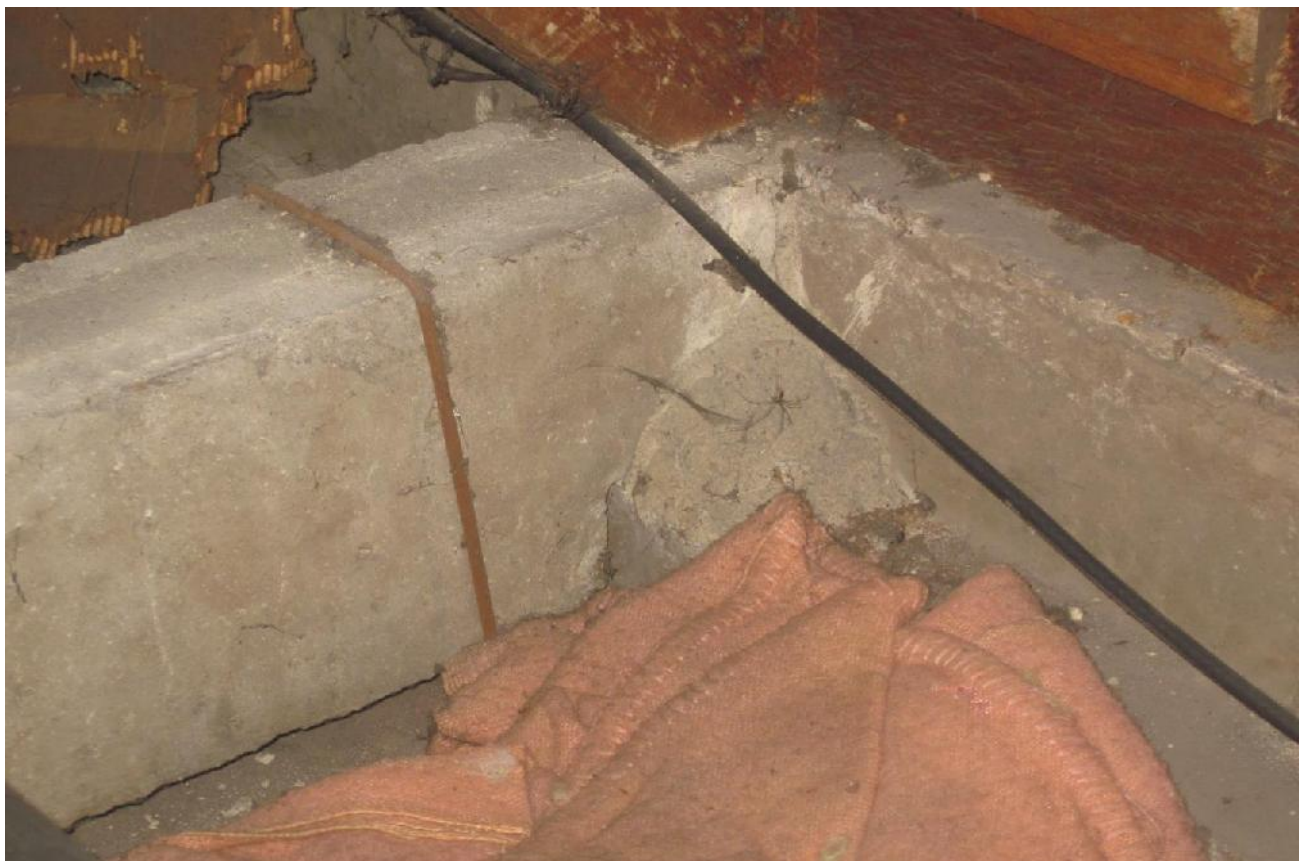
Photograph C11 – Concrete stitch
