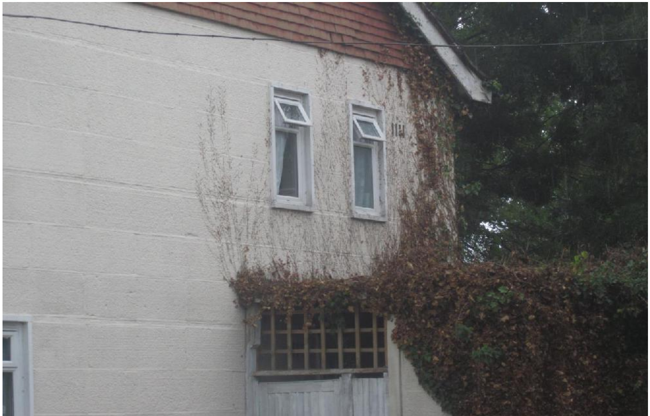
Photograph C24 – Vegetation on elevation
