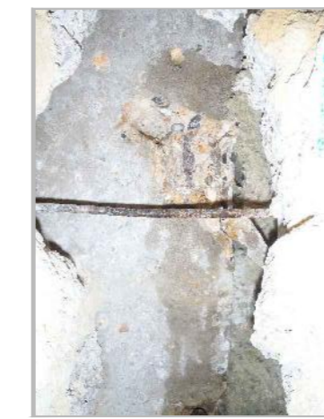
PC6a: VIEW OF B/O C4 TO 1ST FLOOR COLUMN
