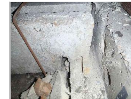
PA3a: VIEW OF SECONDARY BEAM BEARING ONTO PRIMARY BEAM AT SECTION AA-AA POST REMOVAL OF MORTAR HAUNCH
