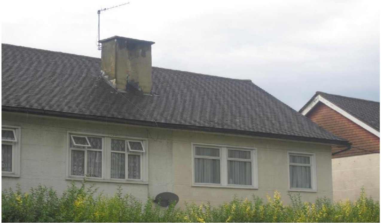
Photograph C26 - Double stack Chimney
