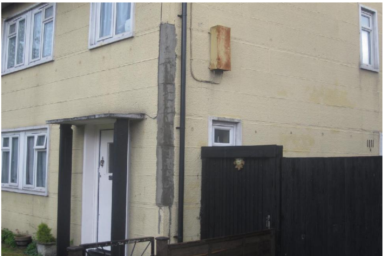
Photograph C17 – Corner cladding patch and repair
