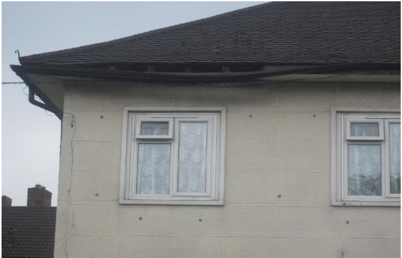
Photograph C28 – Damaged guttering
