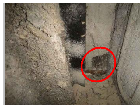
PB11b: VIEW LOOKING DOWN TOWARDS COLUMN BASEPLATE CONNECTION BELOW B/O B5
