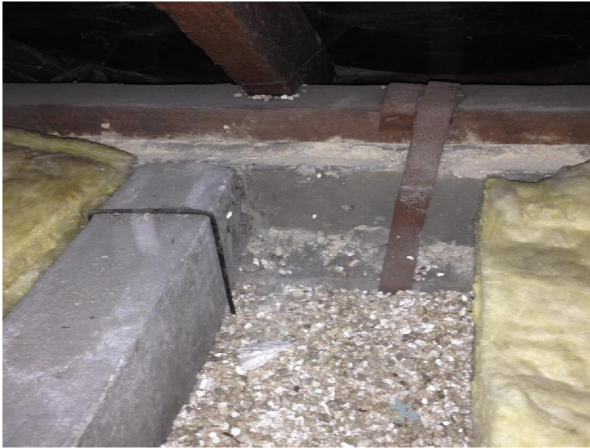
Photograph C5 – Roof sole plate strapping to primary beam
