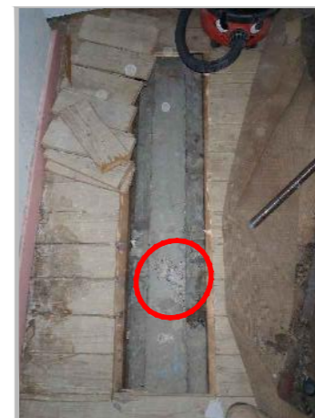
PA10a: GENERAL VIEW OF 1ST FLOOR EXPOSURE AT B/O A4
