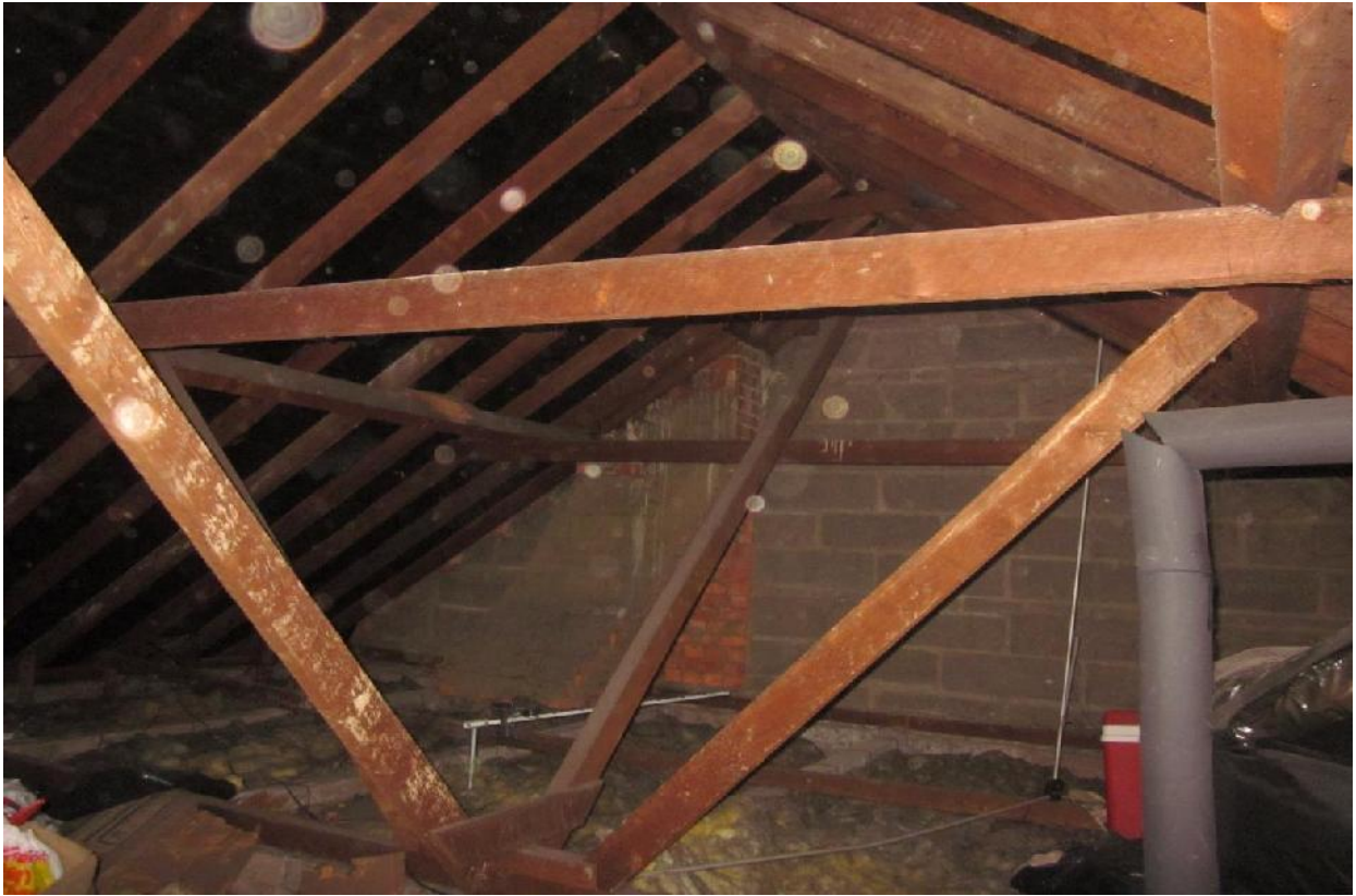
Photograph C14 – 241 Morden Road roof structure
