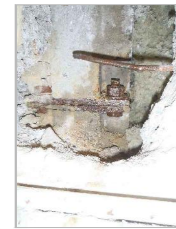
PC6b: VIEW OF 1ST FLOOR TO GROUND FLOOR COLUMN CONNECTION DETAIL
