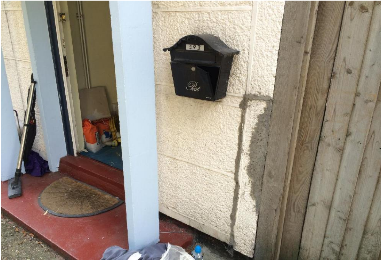
Photograph C30 – Patch repair to corner cladding
