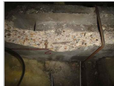
PB4a: VIEW OF BREAKOUT B/O B2 TO TOP OF SECONDARY BEAM
