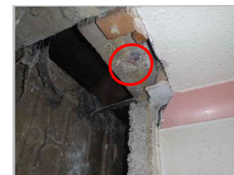
PA6a: GENERAL VIEW OF B/O A3 TO SOFFIT OF PRIMARY BEAM
