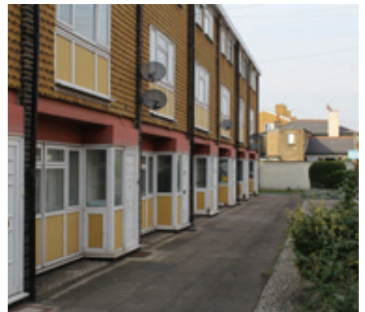
4. Ground floor flats with doors onto the outside, which is an improvement over most of the arrangements elsewhere on site.
