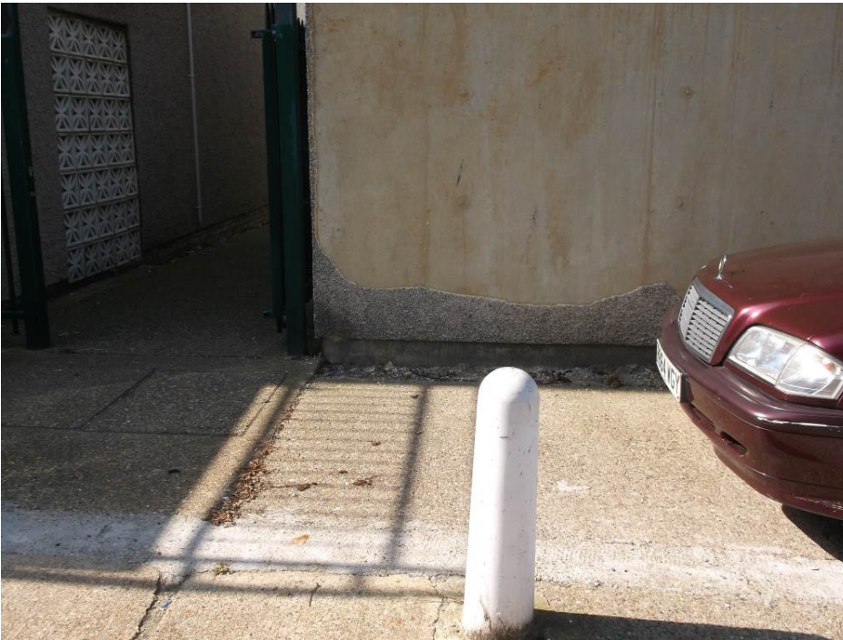
Photograph 8 – Flank wall render removed
