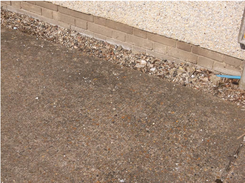
Photograph 4- Base of flank wall
