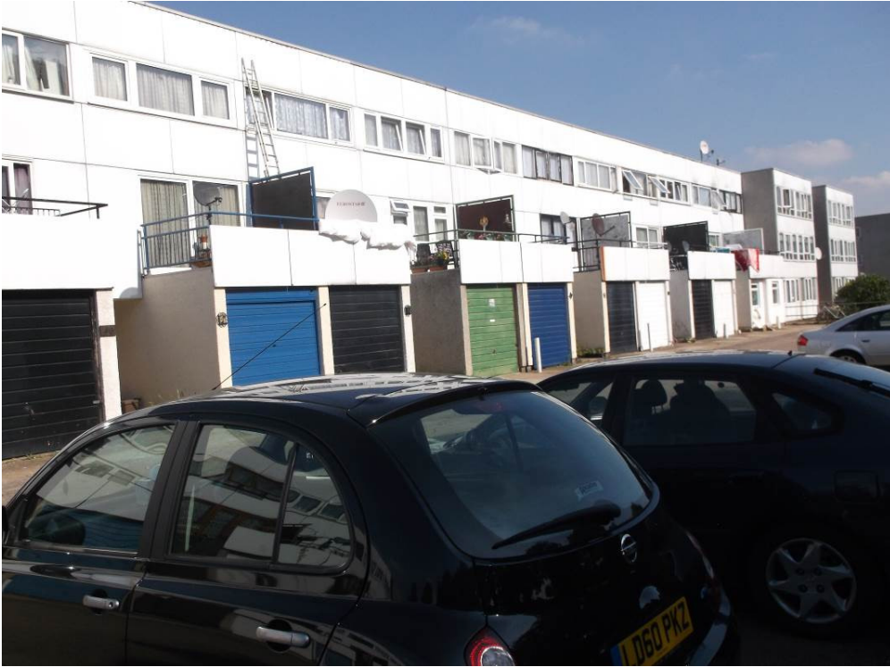
Photograph 1 – Town houses – front elevation
