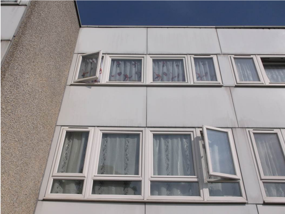
Photograph 13 – Paines Close – Rear elevation
