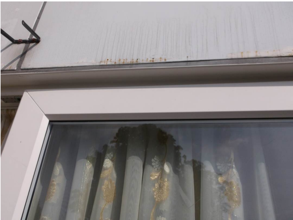
Photograph 14 – 18 Paines Close – Cladding and windows at rear
