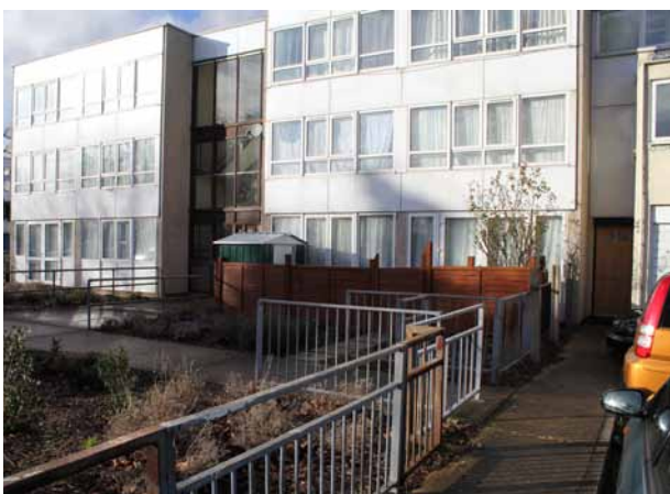
2. The definition between what is public and what is private is sometimes hard to discern, and above, a resident has more clearly defined what is private through the use of a fence.
