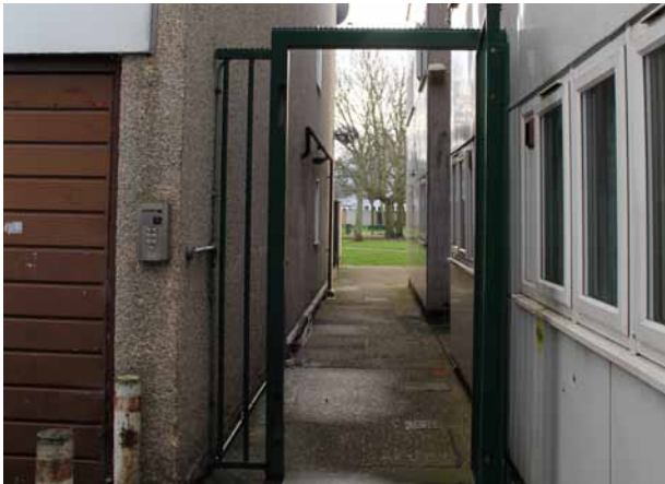
1. Moving from outside the estate to the internal space requires passing through narrow alleyways, all of which were gated but not locked.
