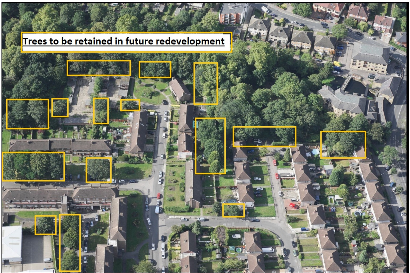
Image above: Trees within the Ravensbury Estate requiring proper survey & retention
