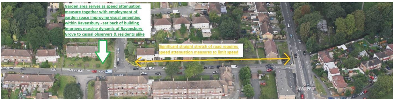
Image above: Northern part of Ravensbury Grove with significant straight stretch of road
