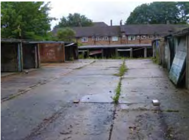
Later addition: Ravensbury garages
