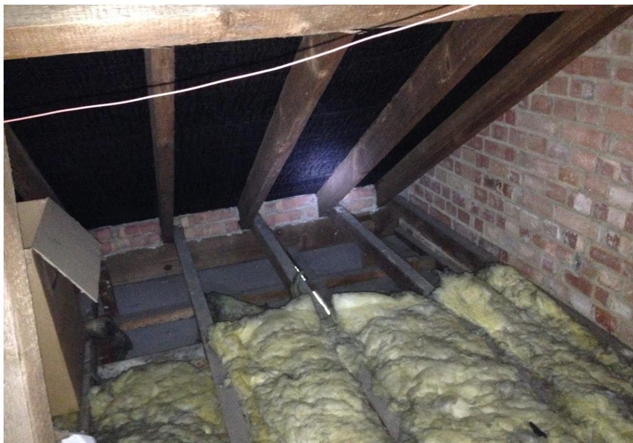
Photograph C8 - 14 Ravensbury Grove Roof Space
