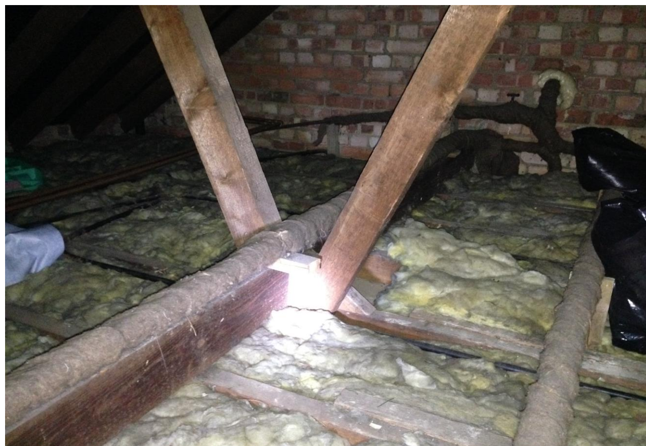
Photograph C10 – 14 Ravensbury Grove Roof Space
