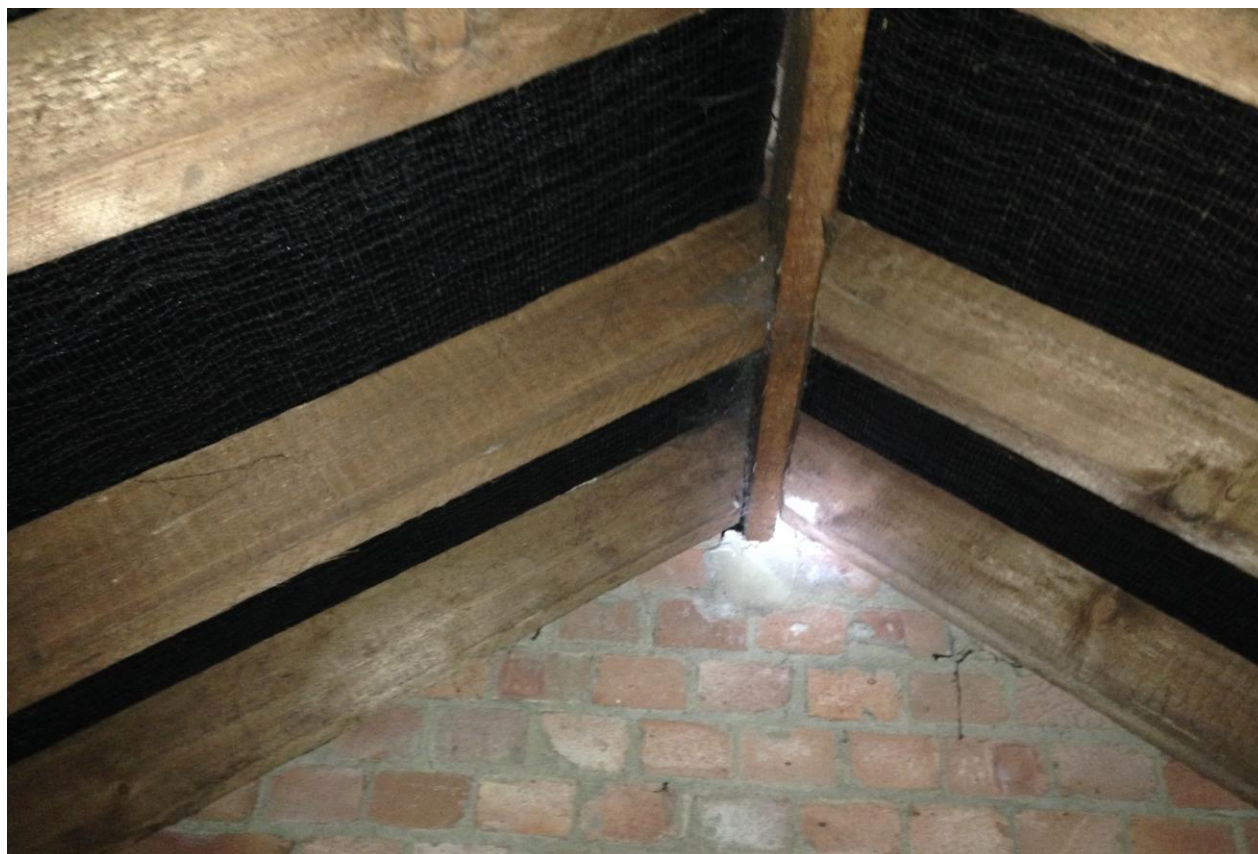
Photograph C7 - 14 Ravensbury Grove Roof Space
