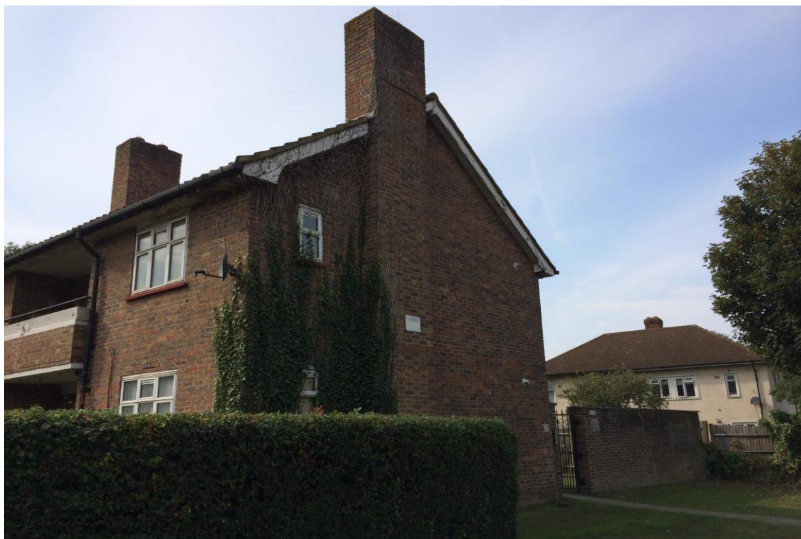
Photograph C12 – Vegetation to Side of Block 4 and Peeling of Paint to Eaves Board
