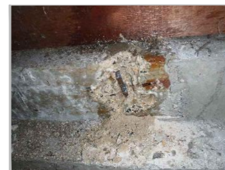
PC4a: VIEW OF B/O C3 TO ROOF PRIMARY BEAM
