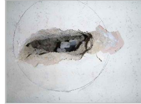
PD8a: VIEW OF B/O D6 AND EXPOSED WALL TIE
