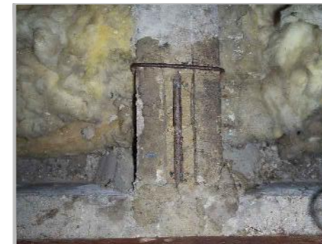
PC2a: VIEW OF B/O C1 TO TOP OF ROOF SECONDARY BEAM
