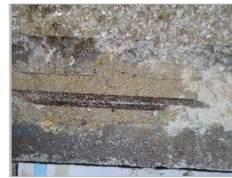
PD2a: VIEW OF B/O D4 TO TOP OF ROOF SECONDARY BEAM
