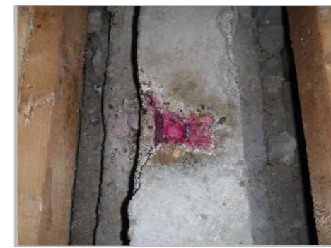
PC7b: VIEW OF B/O C5 TO TOP OF PRIMARY BEAM
