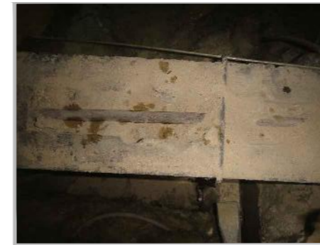
PB2b: VIEW LOOKING DOWN AT BREAKOUT B/O B1
