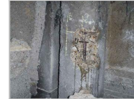
PA8a: VIEW OF B/O A2 TO 1ST FLOOR COLUMN WITHIN CAVITY
