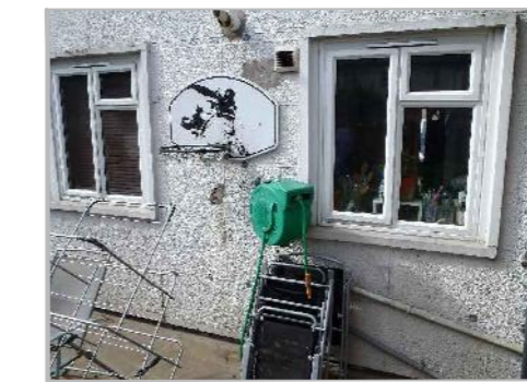
PD13a: PART VIEW OF WALL TIE SURVEY AREA D3
