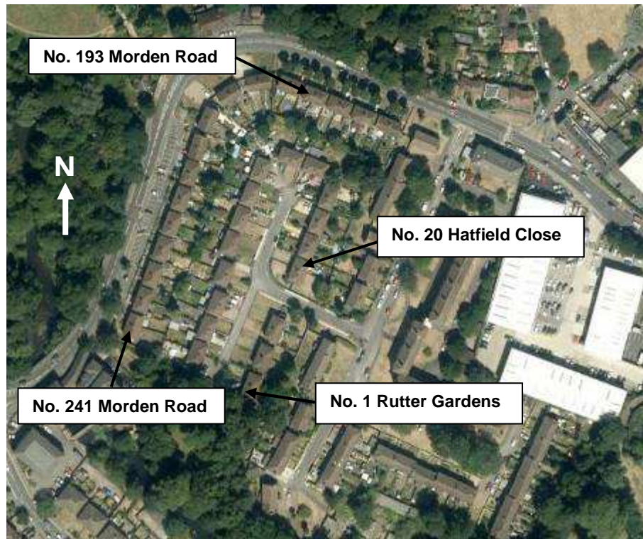
Fig. R1: Aerial view of the Ravensbury Estate showing the position of the four properties investigated
