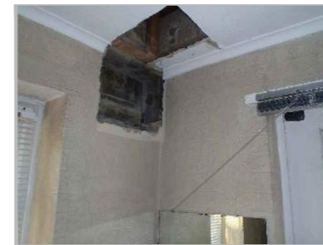
PA9a: GENERAL VIEW OF EXPOSURE EXP A1 IN SOUTH WESTERN CORNER OF PROPERTY
