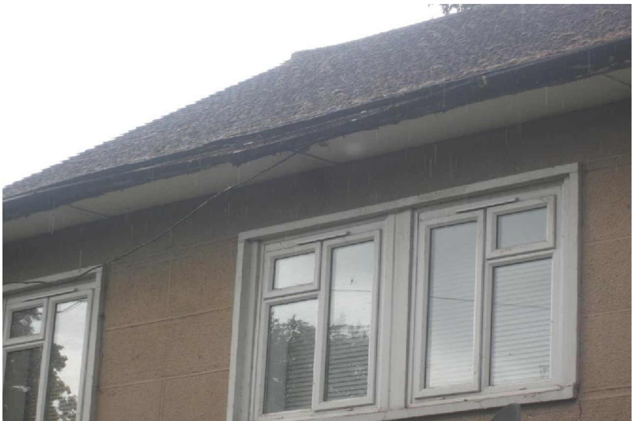
Photograph C29 – Damaged guttering
