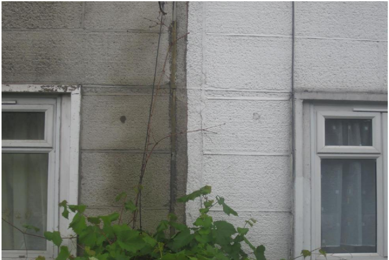
Photograph C22 – Party wall cladding unit mortar repair
