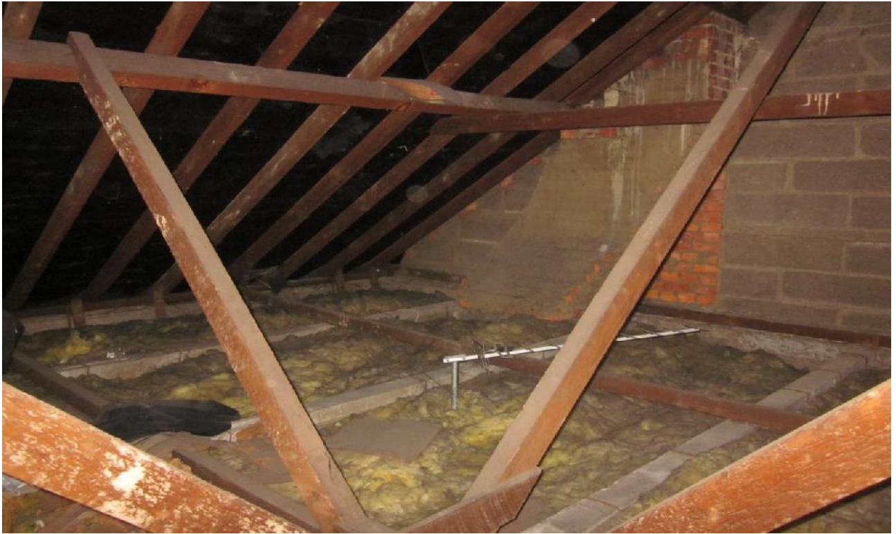
Photograph C12 – 124 Morden Road roof structure
