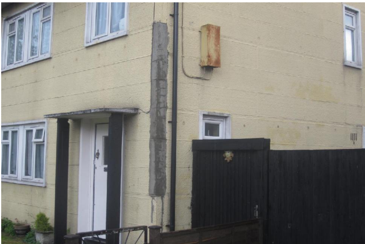
Photograph C17 – Corner cladding patch and repair
