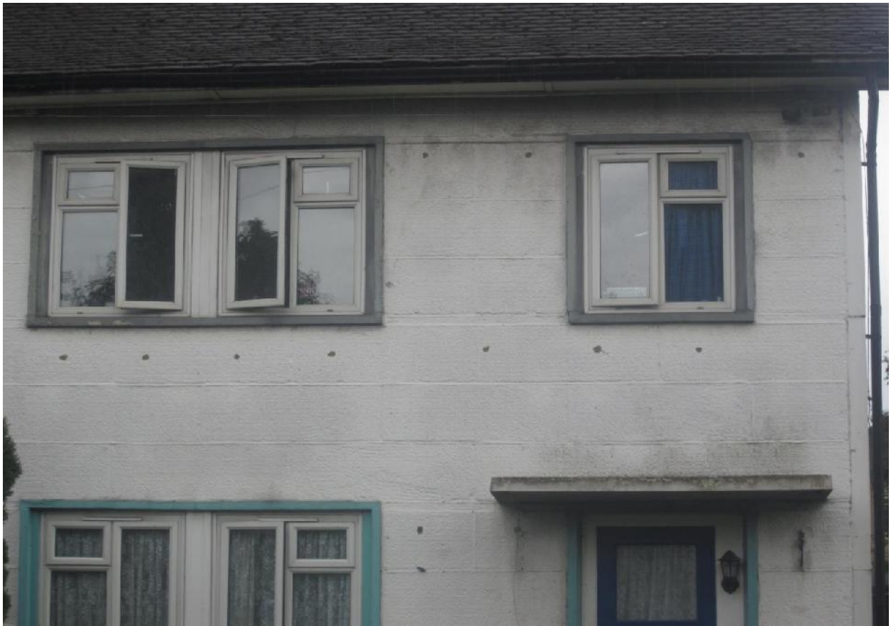
Photograph C18 – Circular markings on elevation
