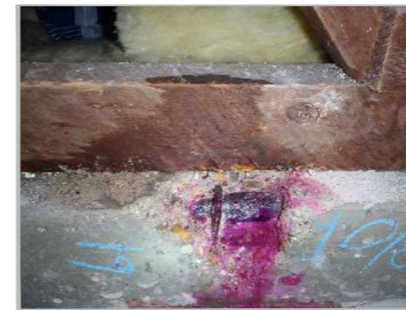
PD3a: VIEW OF B/O D5 TO ROOF PRIMARY BEAM
