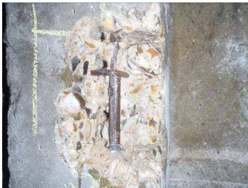
Plate R7: View of column Breakout A2 at No. 241 Morden Road.
