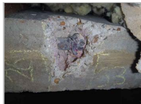
PA5a: VIEW OF B/O A1 TO SOFFIT OF ROOF SECONDARY BEAM
