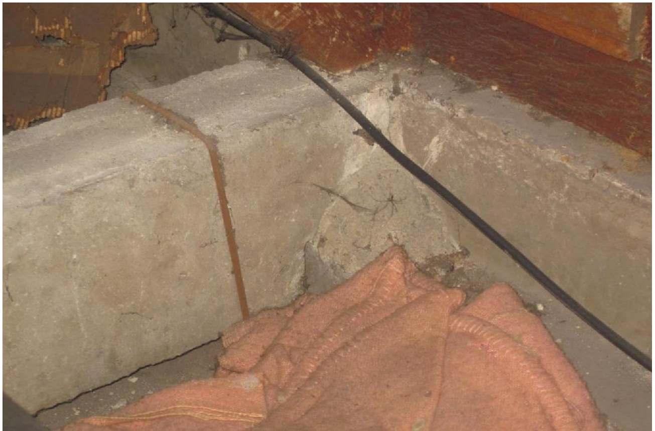
Photograph C11 – Concrete stitch
