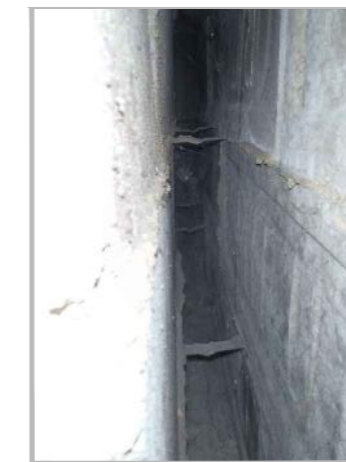
PA11c: VIEW LOOKING SOUTH FROM EXPOSURE EXP A2 WITHIN CAVITY
