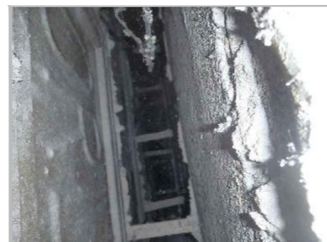
PA5b: VIEW LOOKING DOWN CAVITY ON EASTERN SIDE OF SECONDARY BEAM
