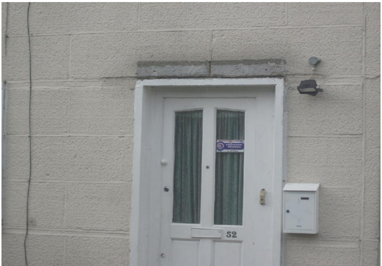
Photograph C25 – Example of removed canopy
