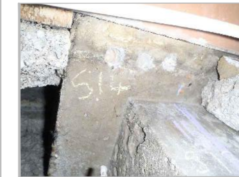
PA11d: VIEW LOOKING UP AT PRIMARY ROOF BEAM BEARING ONTO COLUMN HEAD AT EXPOSURE EXP A3
