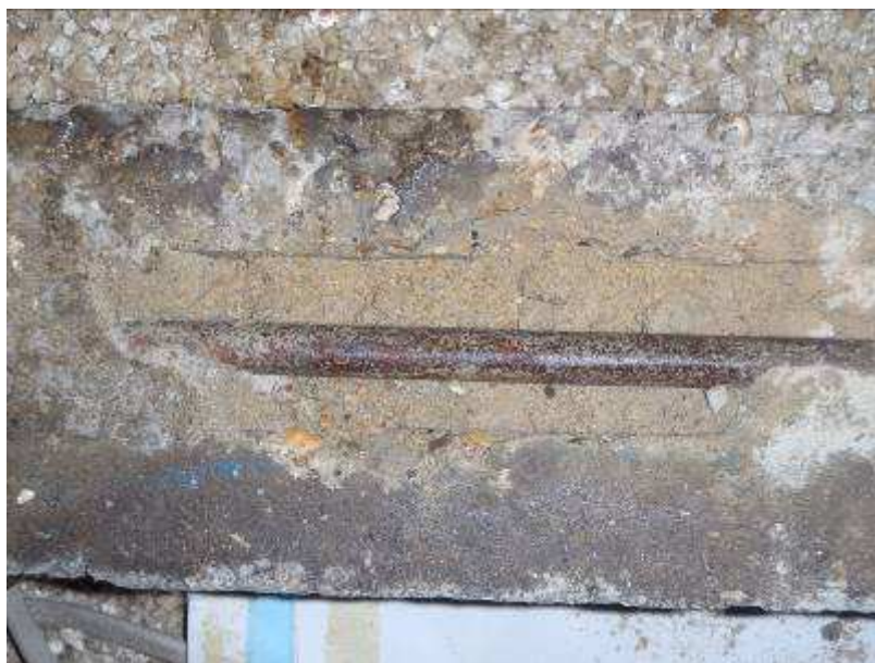
Plate R8: View of Breakout D2 to roof secondary beam continuity bar over central column at No. 20 Hatfield Close.
