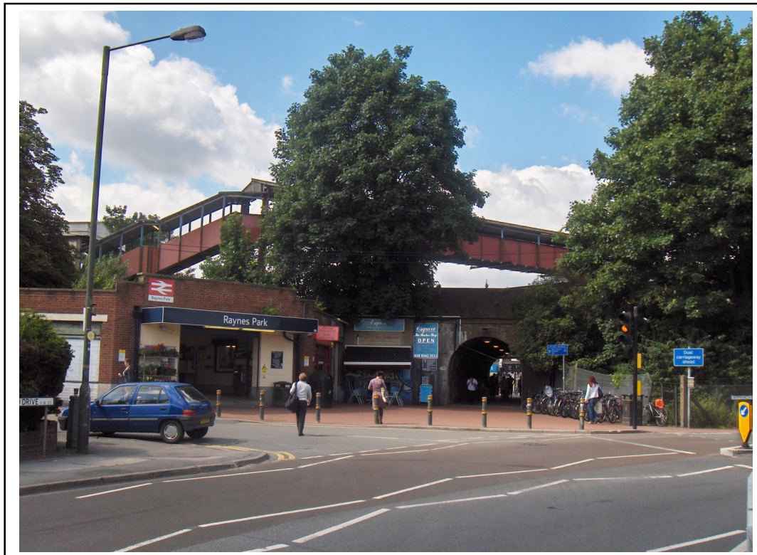
Figure 3 Raynes Park station entrance and Cattle Arch – south side (2013)
