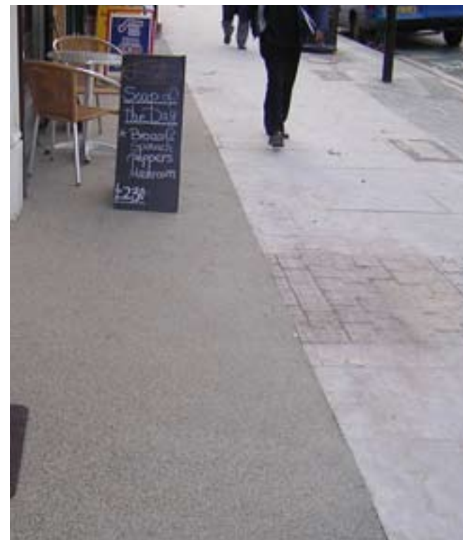
Grey sursert used as for private forecourts, where paving build-up zone is insufficient for paving slabs
