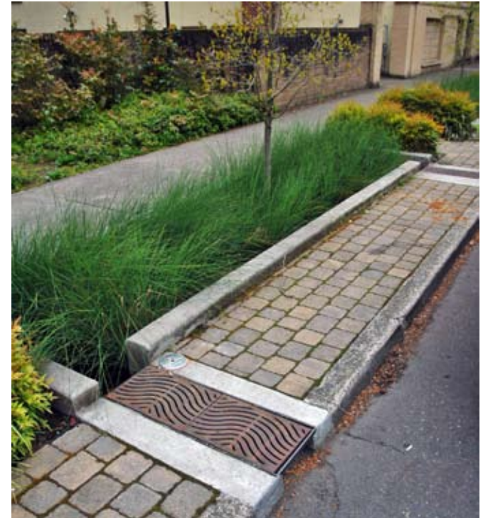
Example of bioretention SUDS in Portland , Oregon
