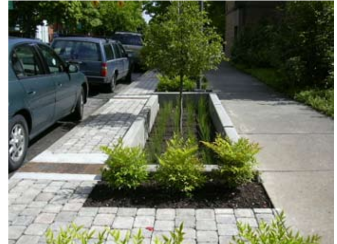
Example of open detention basin SUDS used in a tight urban condition
