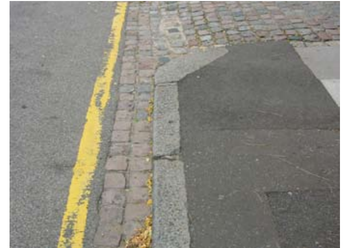
Granite sett channel detail, Wimbledon Village
