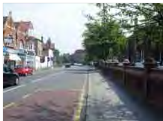
Kingston Road Boundary Wall Section to be retained
