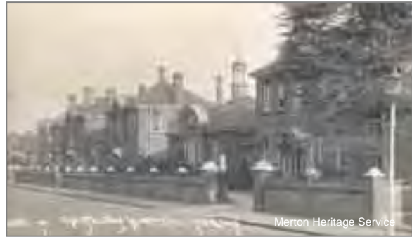
Kingston Road frontage, 1912
