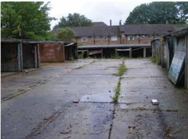
Later addition: Ravensbury garages
