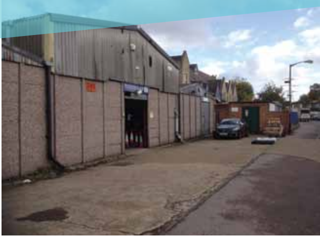
Some buildings on High Path have a negative visual impact
