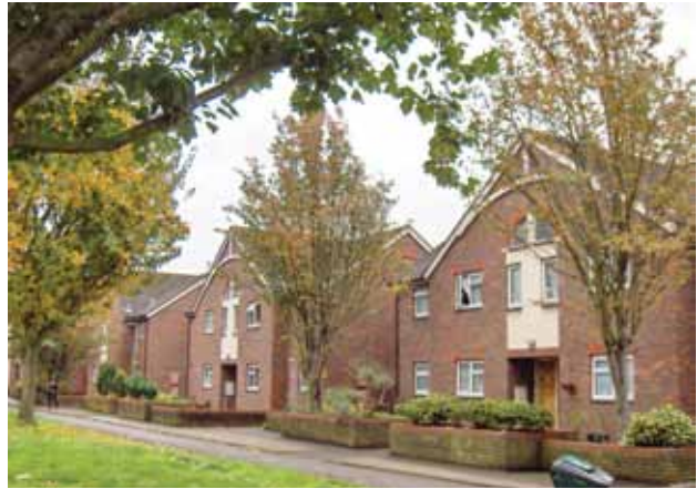
2 storey flats fronting Merton High Street
