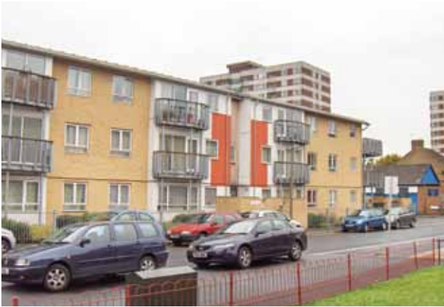
3 storey flats on Nelson Grove Road
