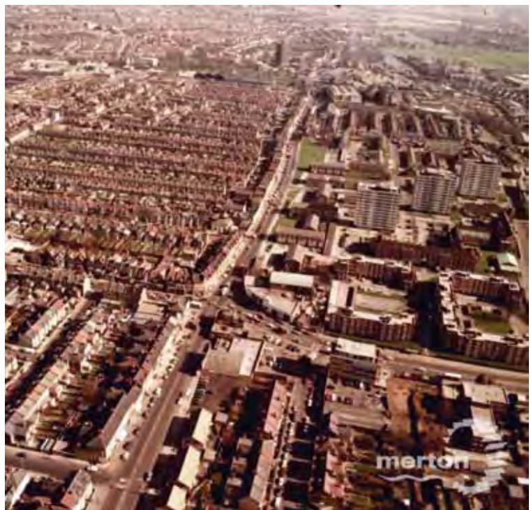
Aerial view Merton High Street - High Path Estate near completion in 1982
