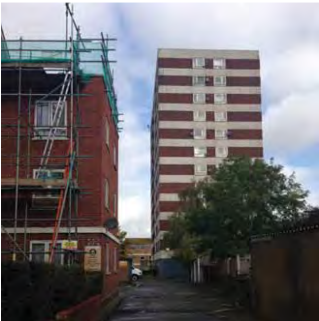
12 storey tower block High Path Estate
