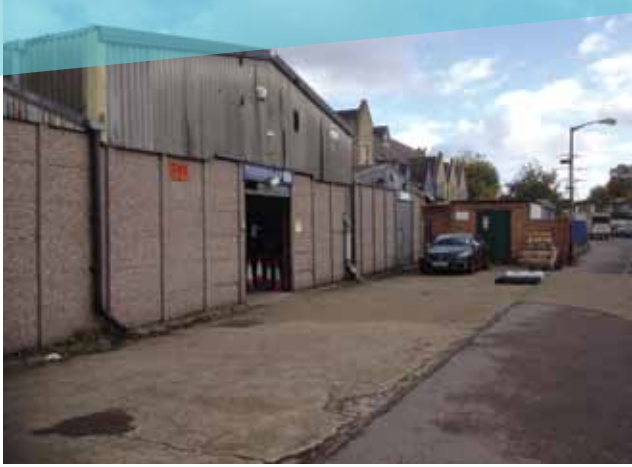
Some buildings on High Path Road have a negative visual impact
