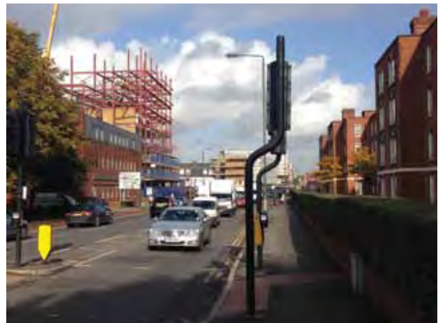
Morden Road (Spur House under construction)
