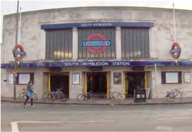
South Wimbledon underground station
