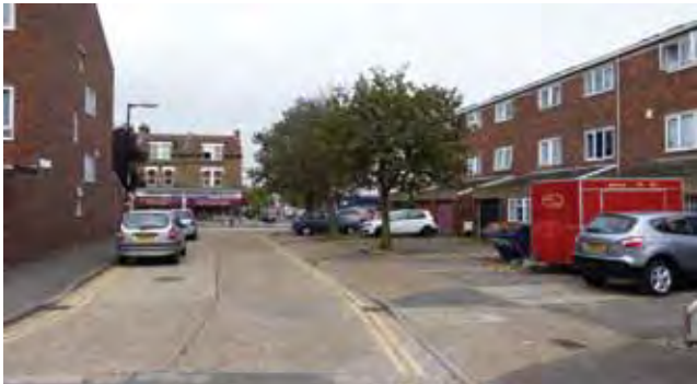
Poorly defined pavements and parking arrangement
