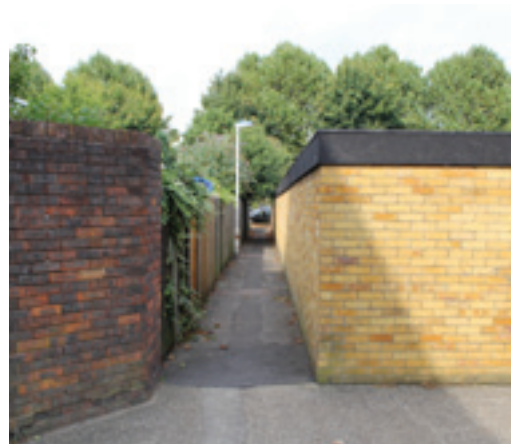
4. Many of the footpaths are narrow and unwelcoming, with poor edges.
