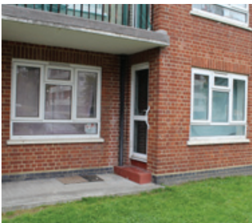
1. Some ground-floor flats offer direct access, but these looked underused.
