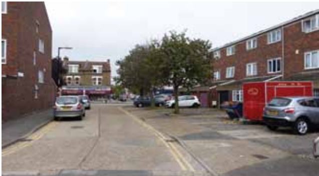
Poorly defined pavements and parking arrangement
