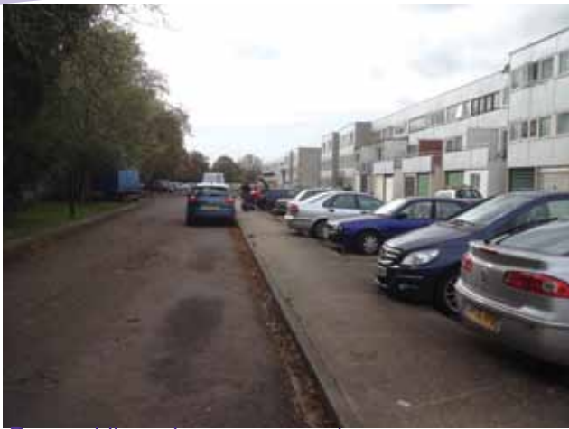
Poor public realm arrangement
