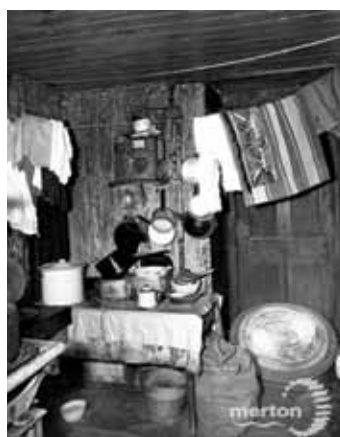
Interior of house in Pincott Road 1961 (prior to demolition)
