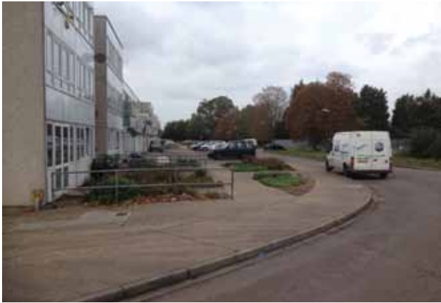
Ill defined space around perimeter of the estate
