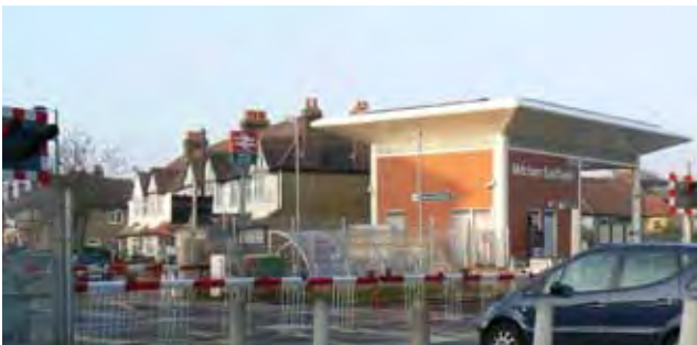
Level crossing at Mitcham Eastfields station
