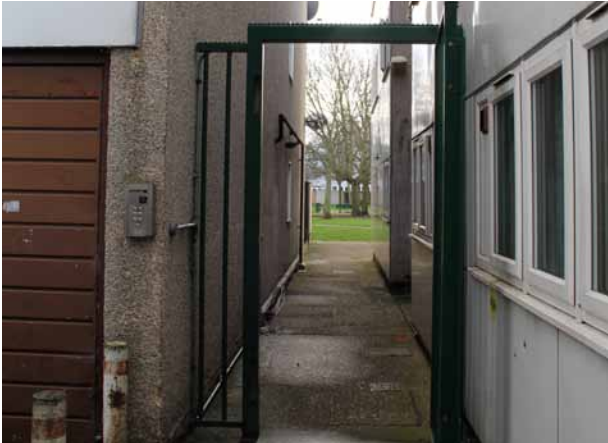
1. Moving from outside the estate to the internal space requires passing through narrow alleyways, all of which were gated but not locked.
