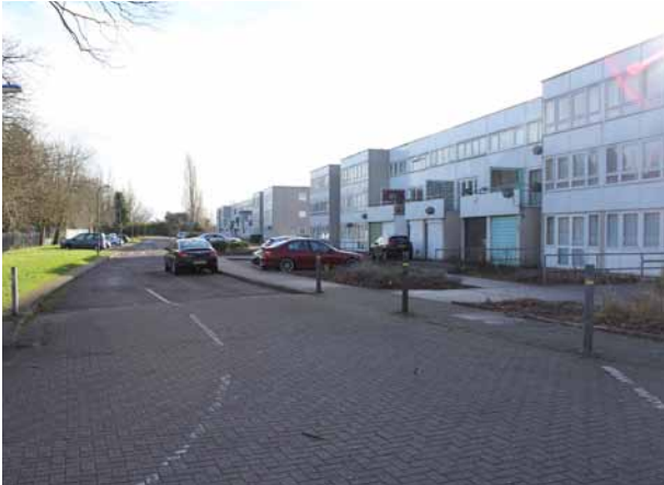
1. The corner of Mullholland Close and Clay Avenue uses block paving to help calm traffic. The rest of the estate uses standard road types and materials.
