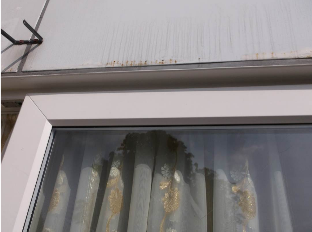
Photograph 14 – 18 Paines Close – Cladding and windows at rear
