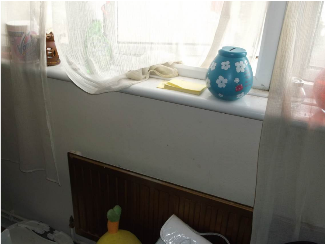
Photograph 11 – Typical panel below windows in flats
