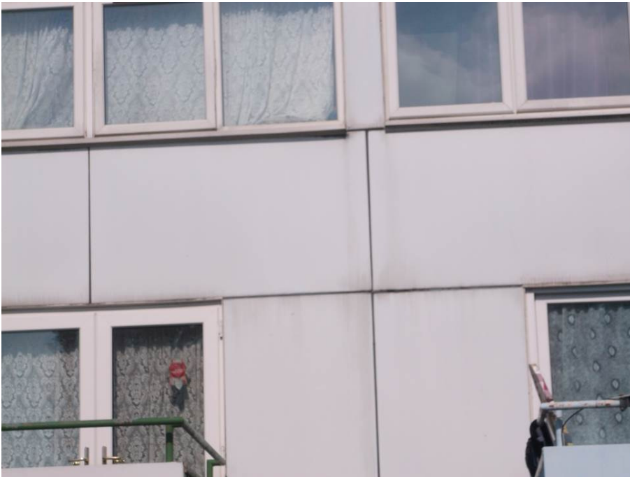
Photograph 3 –Typical cladding to flats
