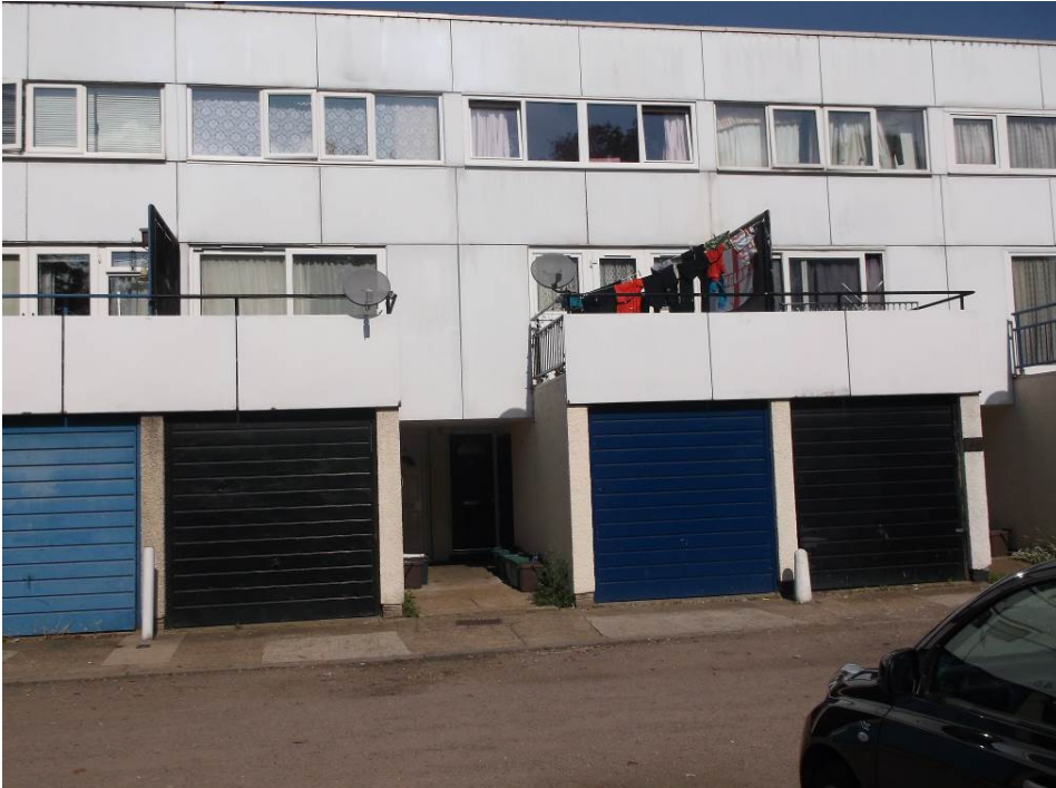
Photograph 2 – Town houses – front elevation
