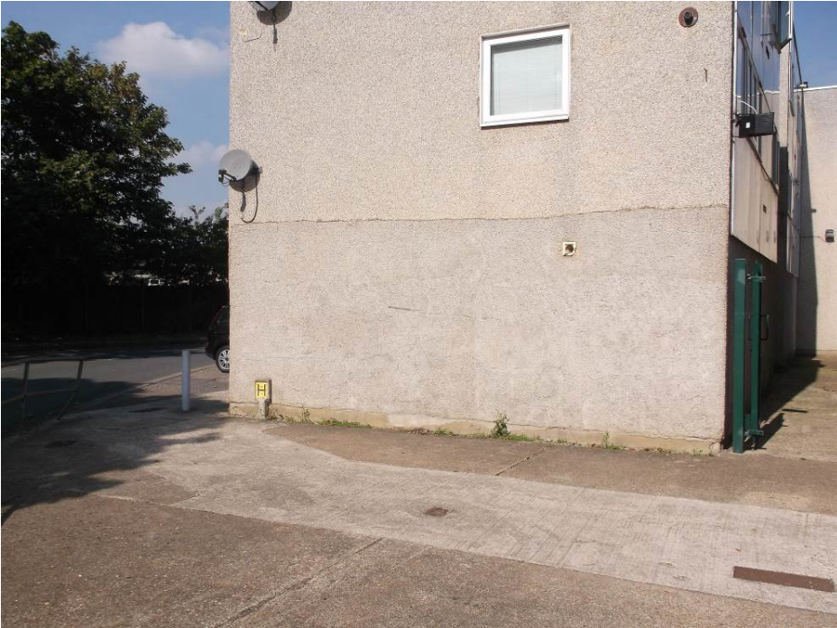
Photograph 9 – Flank wall rendered
