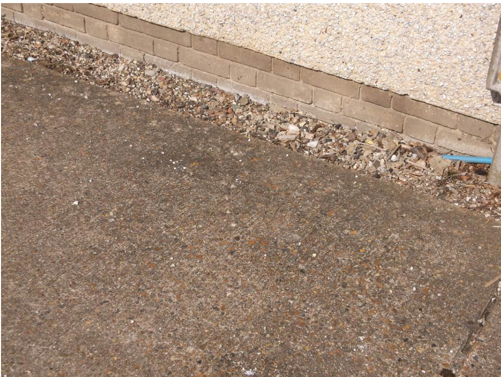
Photograph 4- Base of flank wall
