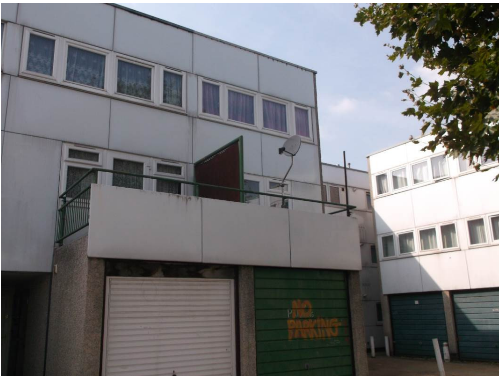
Photograph 12 – Front elevation 18 Paines Close
