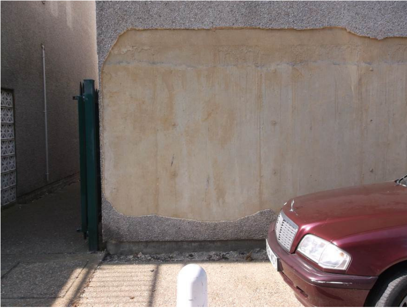
Photograph 7 – Flank wall render removed
