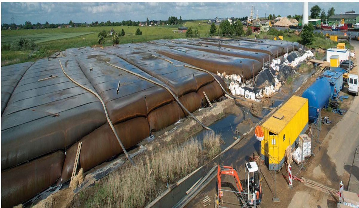
Silt bags being used to store silts until the material has dried and become more stable.
