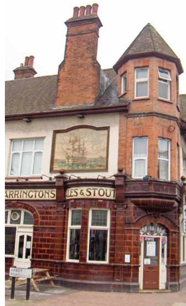
The Nelson Arms marks the site of the entrance gates into Merton Place
