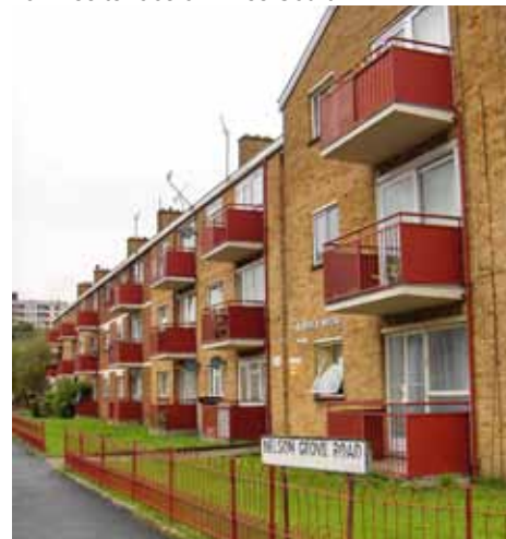
Cantilever balconies on Nelson Grove Road
