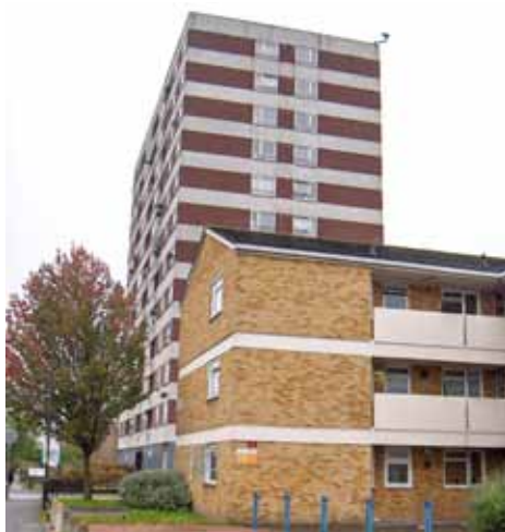
3 storey block and 12 storey tower on Pincott Road
