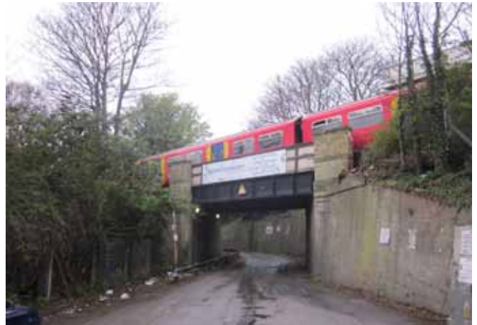
Photograph 14: Under bridge access to site
