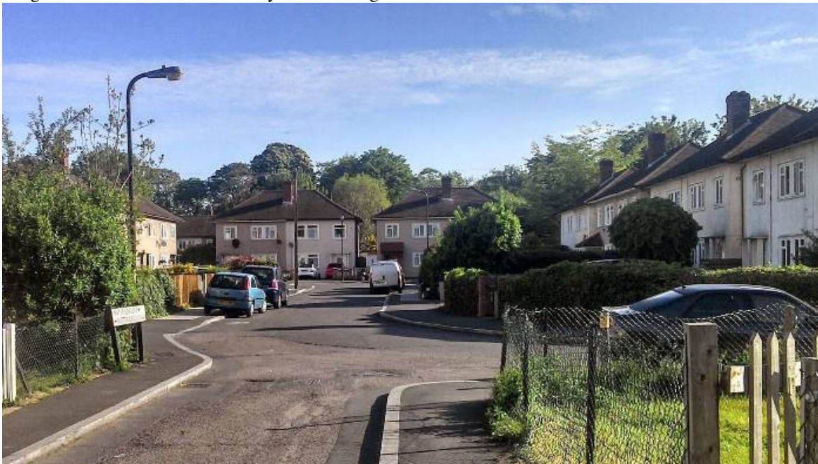
Image above: View along Hatfeild Close with tree-line including Morden Hall Park beyond.
