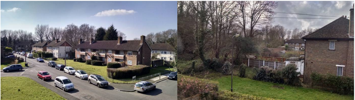
View across Ravensbury Grove (LHS) & View behind Hengelo Gardens towards garages area (RHS)
