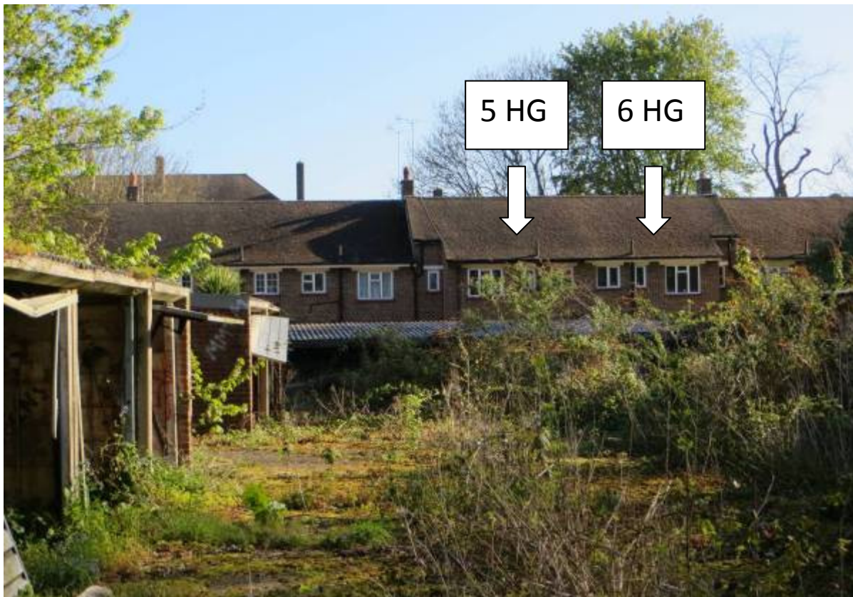
View from within the currently derelict garages site, looking towards Hengelo Gardens with the roof to the 4 storey section of Ravensbury Court visible beyond. Height difference between the derelict garages area & the houses on Hengelo Gardens beyond can be appreciated here.
