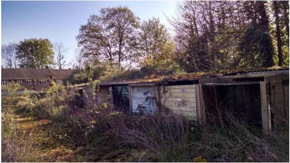
Derelict garages site indicating existing scale
