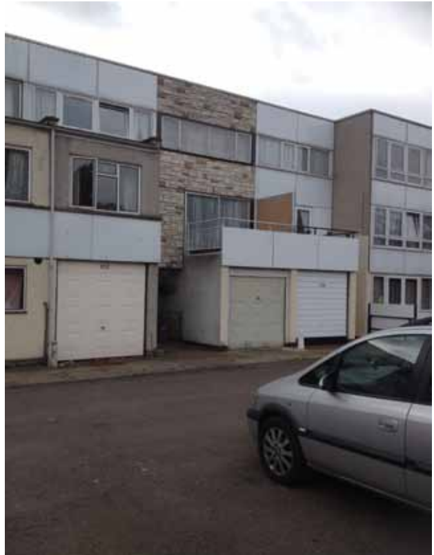
Garage doors dominate ground floor frontages
