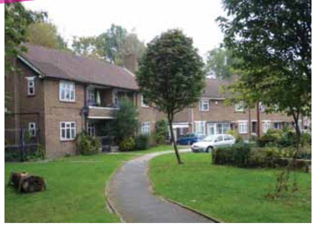
South end of Ravensbury Grove
