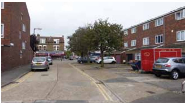
Poorly defined pavements and parking arrangement
