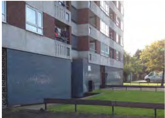
Unclear communal entrance with blank street frontage
