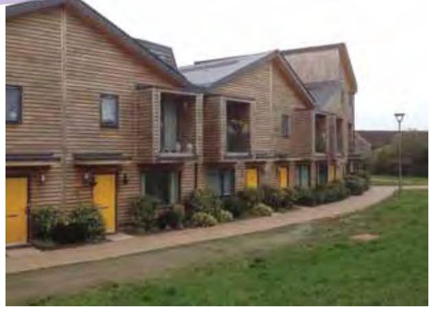
2 storey houses at Rowan Park
