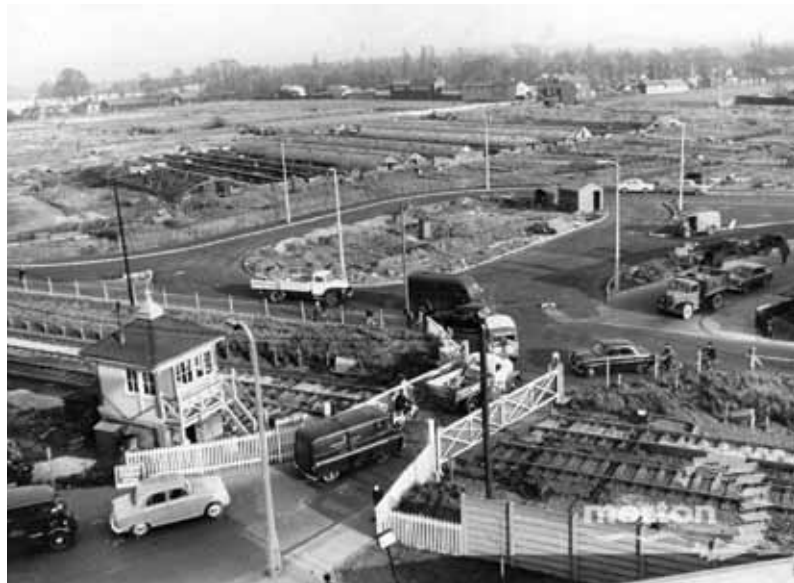
Eastfields level crossing 1961
