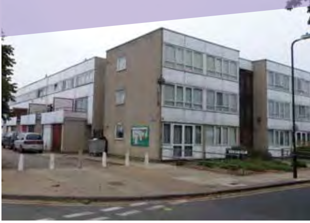
3 storey apartment blocks Eastfields
