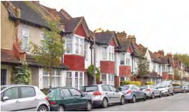
Character area 2: Mill Road
