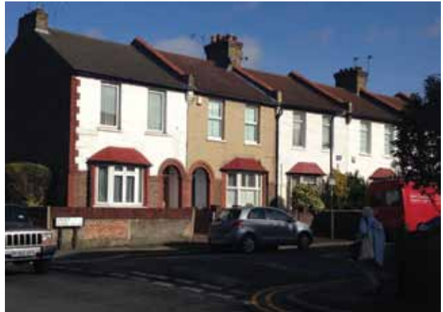
Residential use on Croft Road
