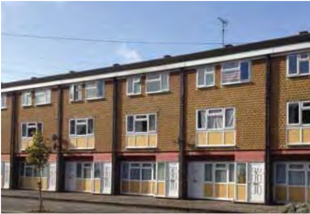
Lack of defensible space
