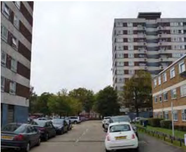
Rear of building block along street frontage
