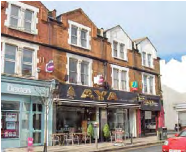
3 storey buildings fronting Merton Road
