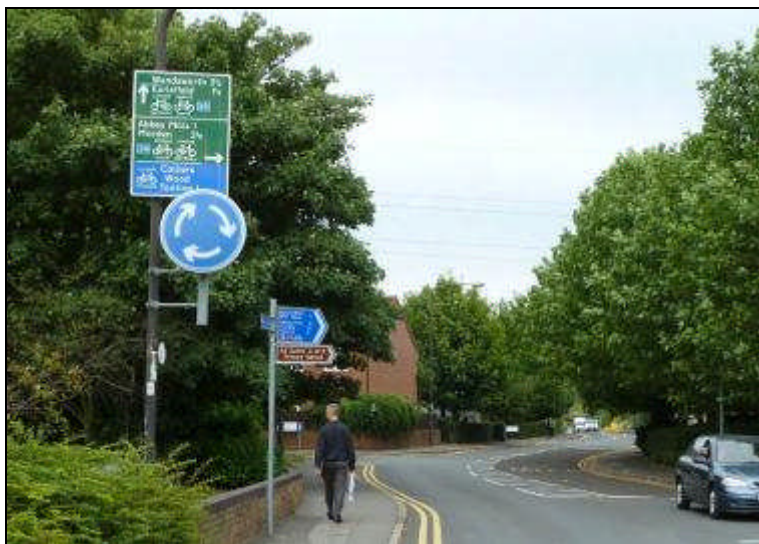
North Road – excessive signing (and incorrect background colour)
