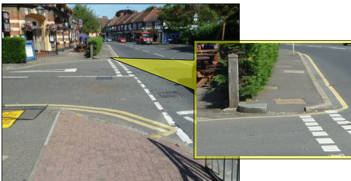
Crossing CR778 Merton Hall Road junction with Kingston Road Dropped kerb on one side only or using driveway/access
