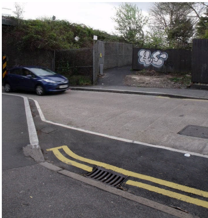
Crossing CR770 Railway Path / Lower Downs Road
