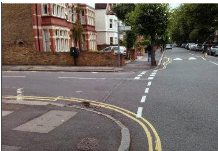
Crossing CR447 Avebury Road junction with Merton Hall Road
