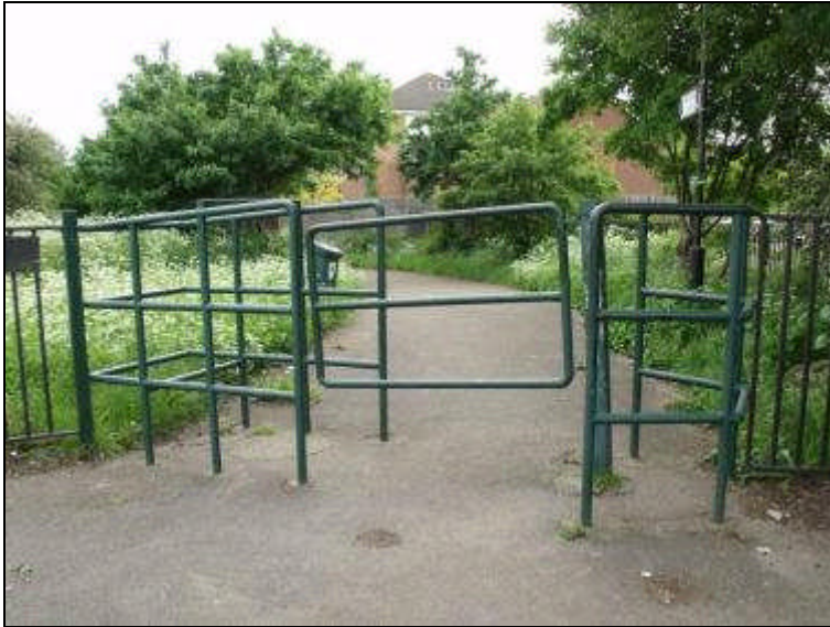
Entrance to path off Fleming Mead (signed as cycle route)
