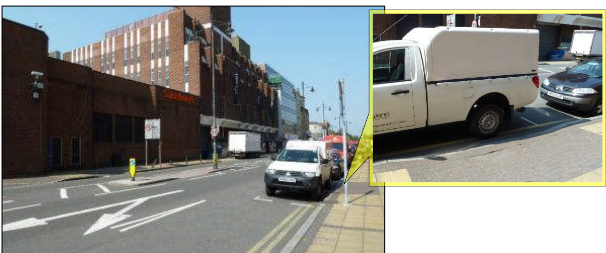
CR753 St George's Road – crossing with dropped kerbs & wide island blocked by parking bay
