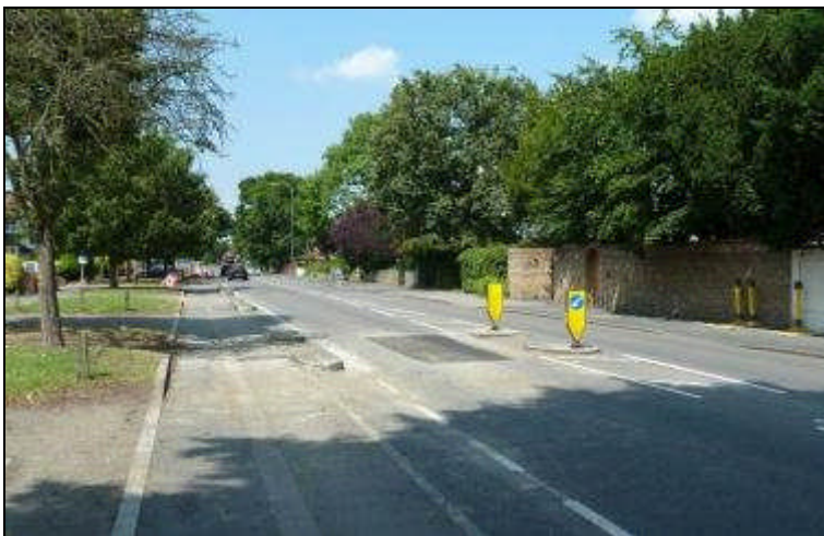
Crossing CR507 Coombe Lane (1.2m refuge plus very narrow kerb between cycle track & road)
