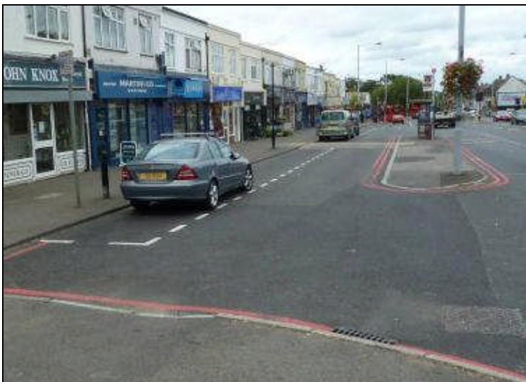
Crossing CR382 Stonecot Hill service road south of junction with Tudor Drive
