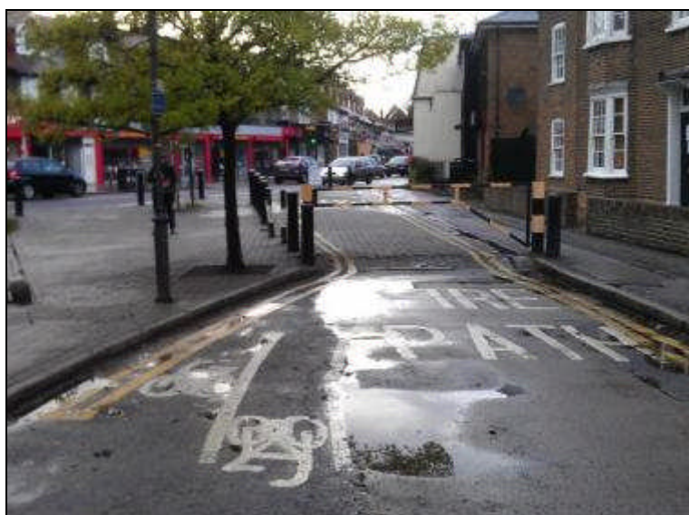
Gated closure of western end of Commonsie East
