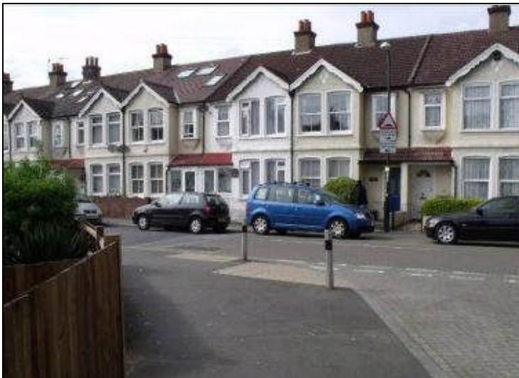
CR073 St Mark's Road junction with Baker Lane – crossing of raised table blocked by parking
