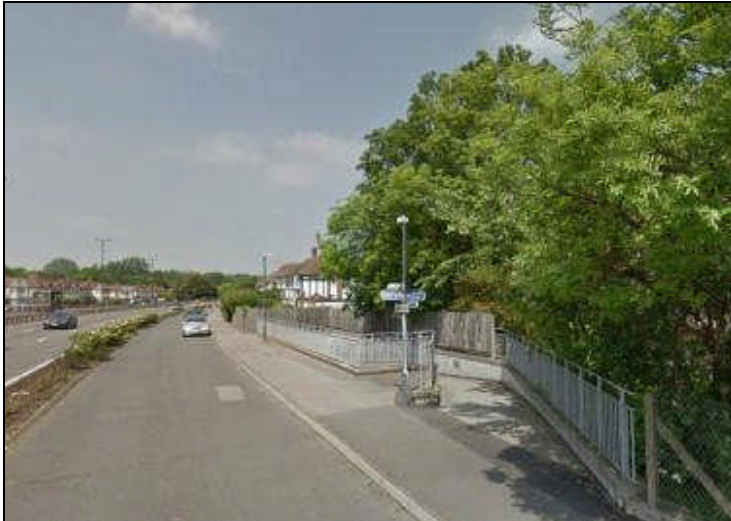
Ramp at eastern end of Westcoombe Avenue subway under A3 (CR500)
