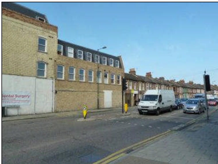
Crossing CR627 Haydon's Road junction with Merton High Street – tactiles on footways but not at refuge
