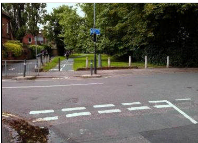
Crossing CR451 Merton Hall Road opposite junction with Henfield Road – end of cycle track but no crossing for pedestrians
