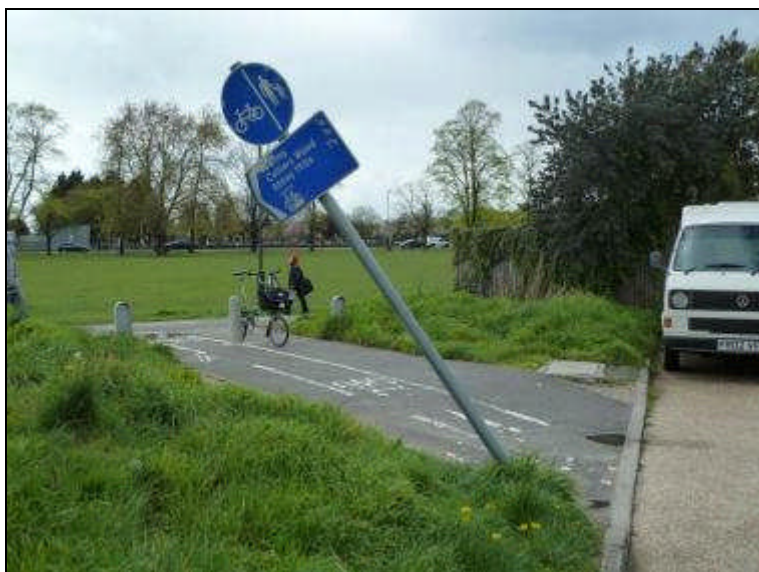
Fig's Marsh – damaged (and unclear) signing
