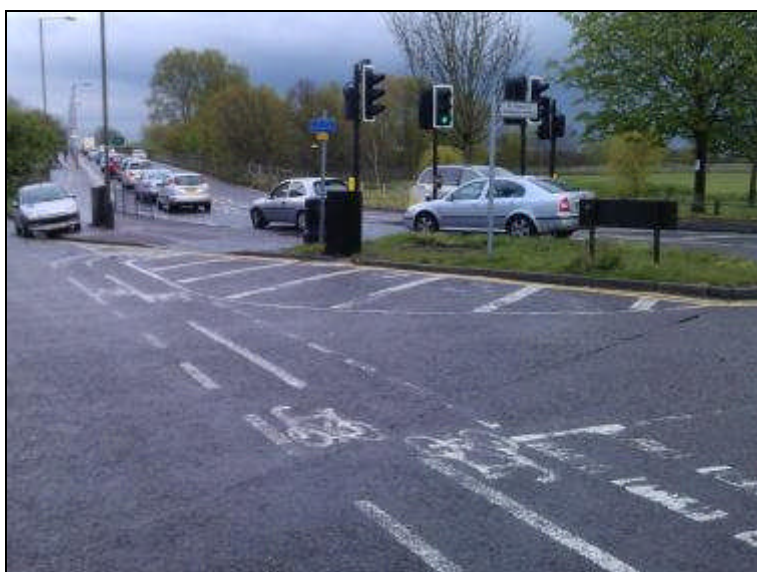
Toucan crossing CR219 across the main section of Commonside East
