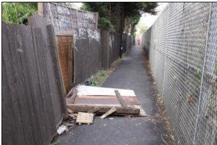
Damaged fencing, Railway Path
