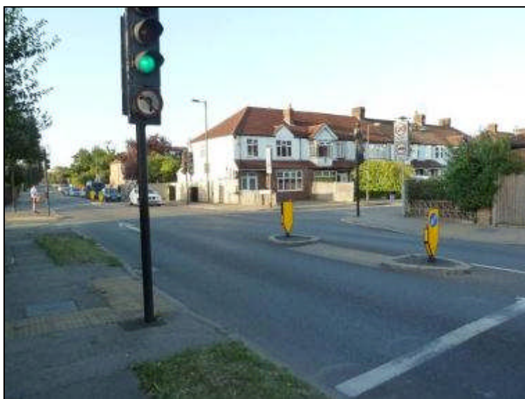
Crossing CR842: Grand Drive south of junction with Crossway, with narrow refuge
