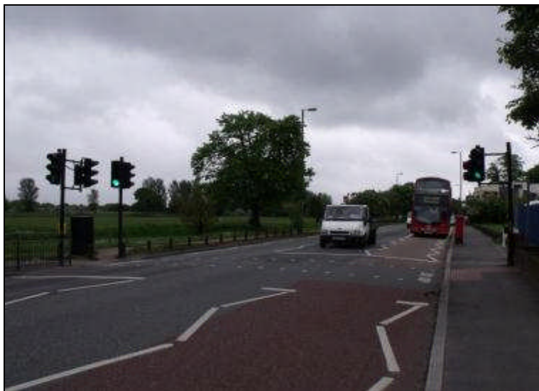
Pelican crossing CR209 of Commonside West
