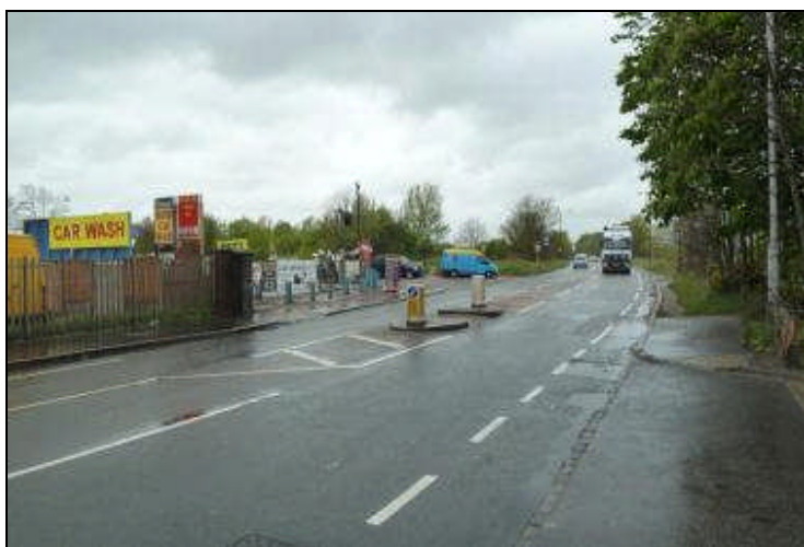
Crossing CR209 of Croydon Road south of eastern edge of Mitcham Common
