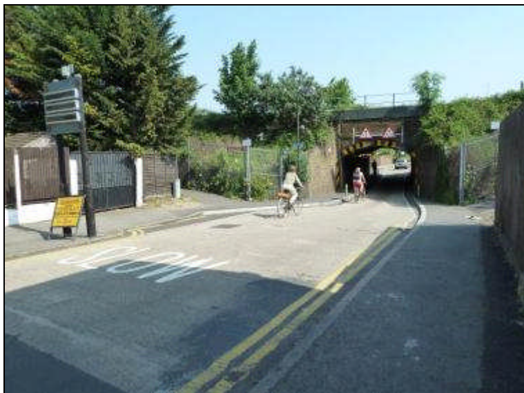
Tunnel under railway, Lower Downs Road
