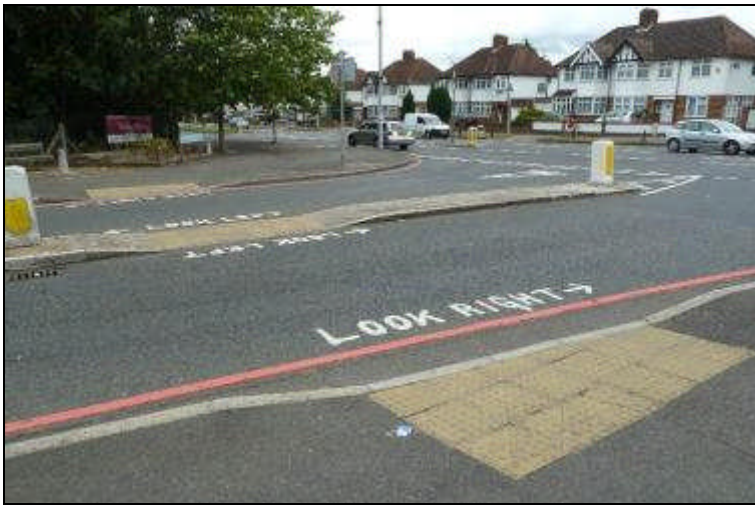
Crossing CR373 Lower Morden Lane junction with Epsom Road (1.2m refuge in reservation)
