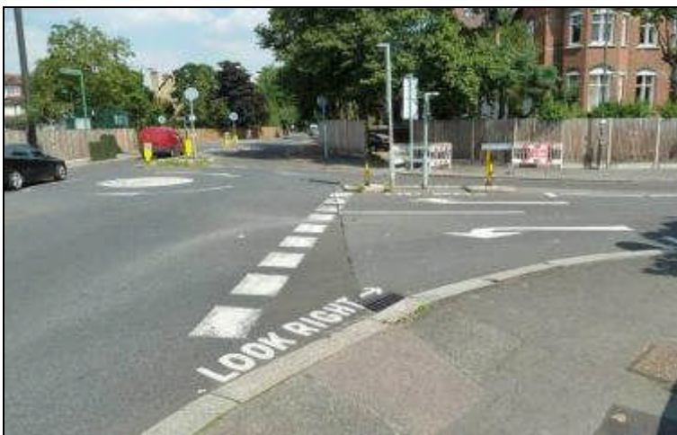
CR536 Cottenham Park Road junction with Cope Hill – refuge not aligned with dropped kerbs on footway
