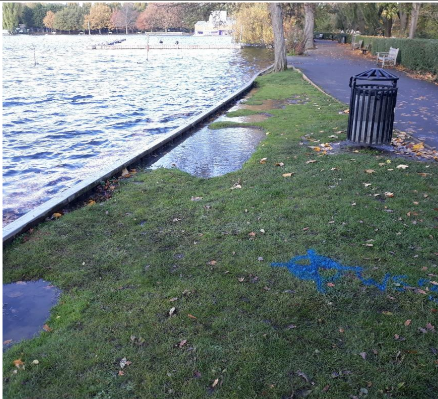
Plate 20 General view of sheet piles looking north. Note: piles in this area stand proud of the retained material and loss of section to the piles permits water to pass through and pond behind.
