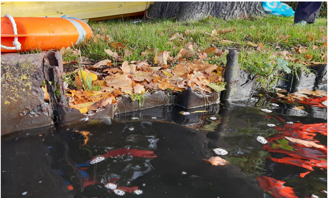
Plate 24 Degredation of the sheet pile on fishing bank
