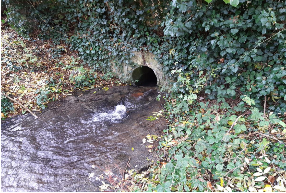
Plate 19 Outfall of the culvert draining the stilling pond
