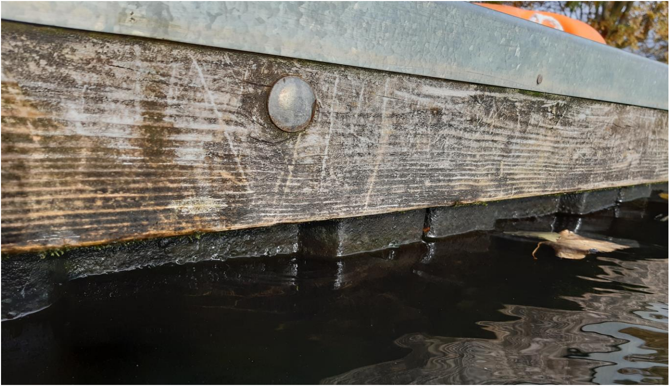
Plate 7 Timber fender strip with metallic capping
