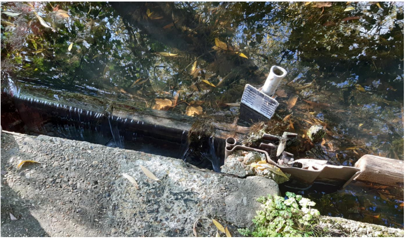
Plate 17 Lake overflow stoplogs
