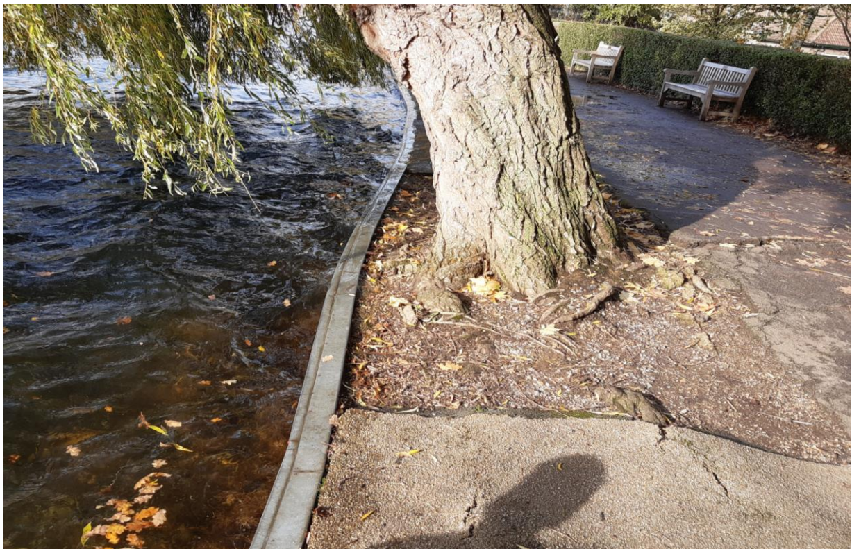
Plate 12 Bulging of the sheet pile due to trees in the central east area of the site
