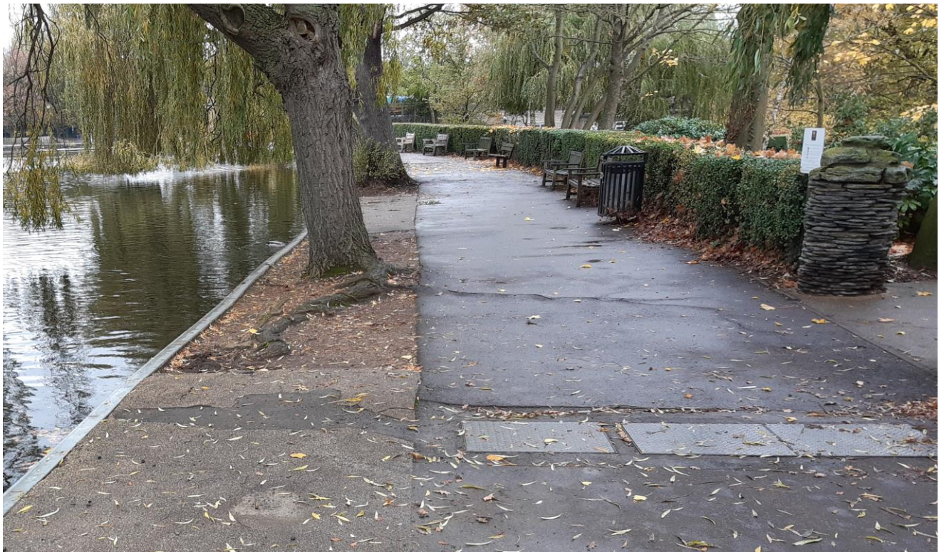
Plate 10 Undulations in the asphalt due to root balls in the central east area of the site
