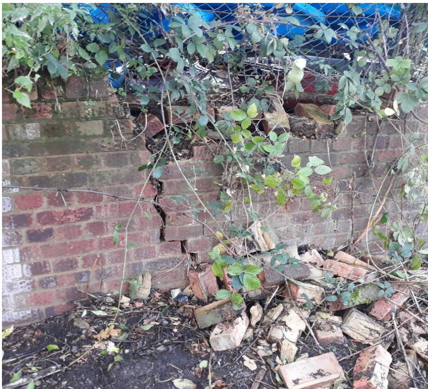
Plate 26 Structural Crack running the full visible height of the brickwork retaining wall
