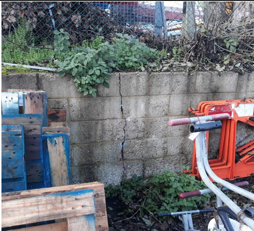
Structural crack running the full height of the blockwork wall
