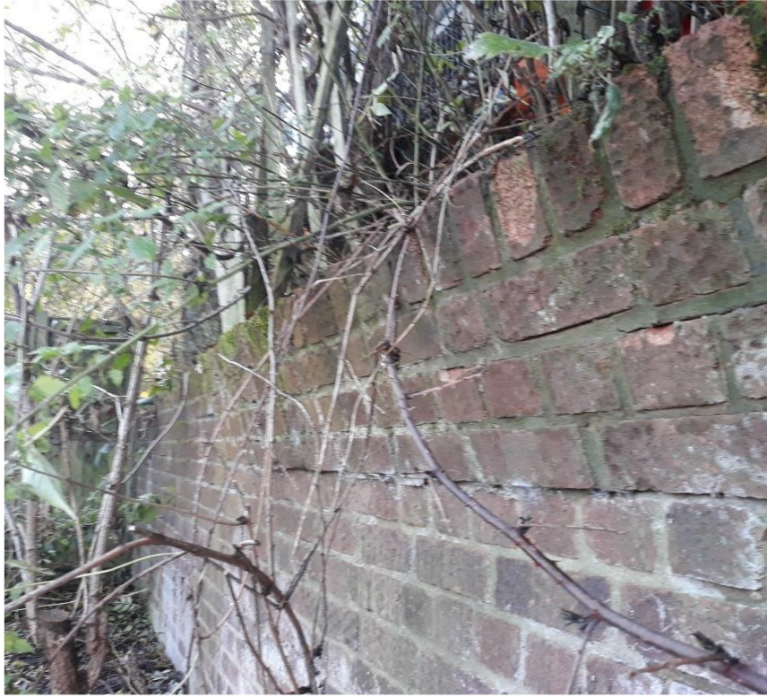
Top section of brickwork retaining wall rotated about a failure plain along a mortar joint
