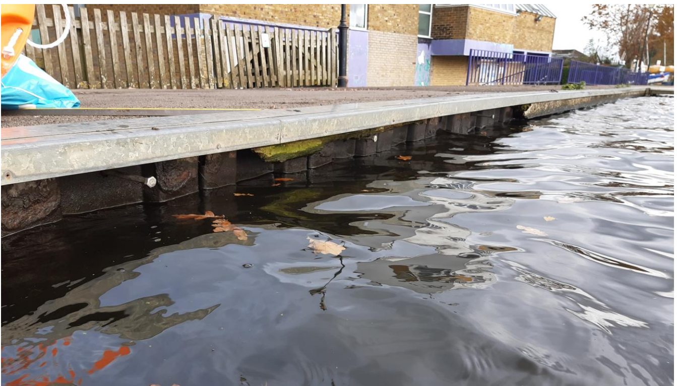
Plate 8 Degredation of the timber fender/rubbing strip in the foreground
