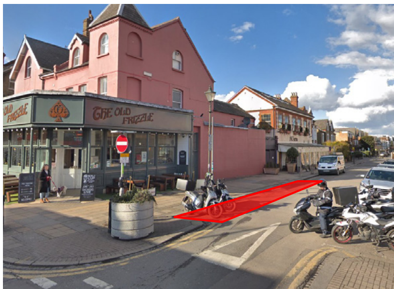
Location of parklet structure highlighted in red
