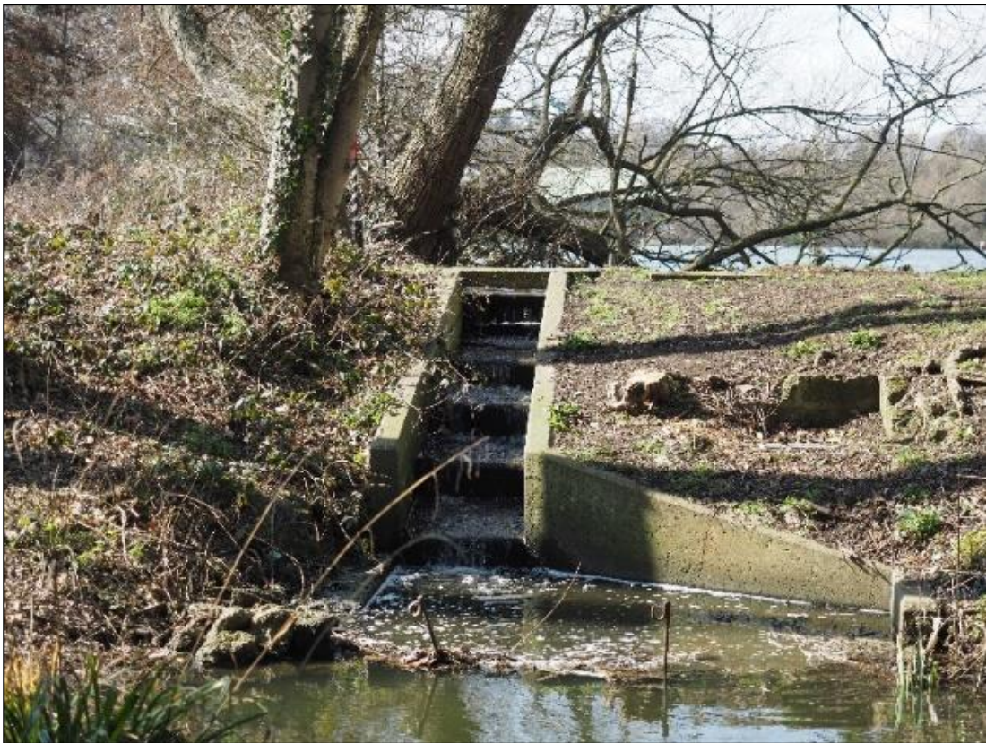
Figure 1.2: Overflow Weir Structure from Wimbledon Park Lake
