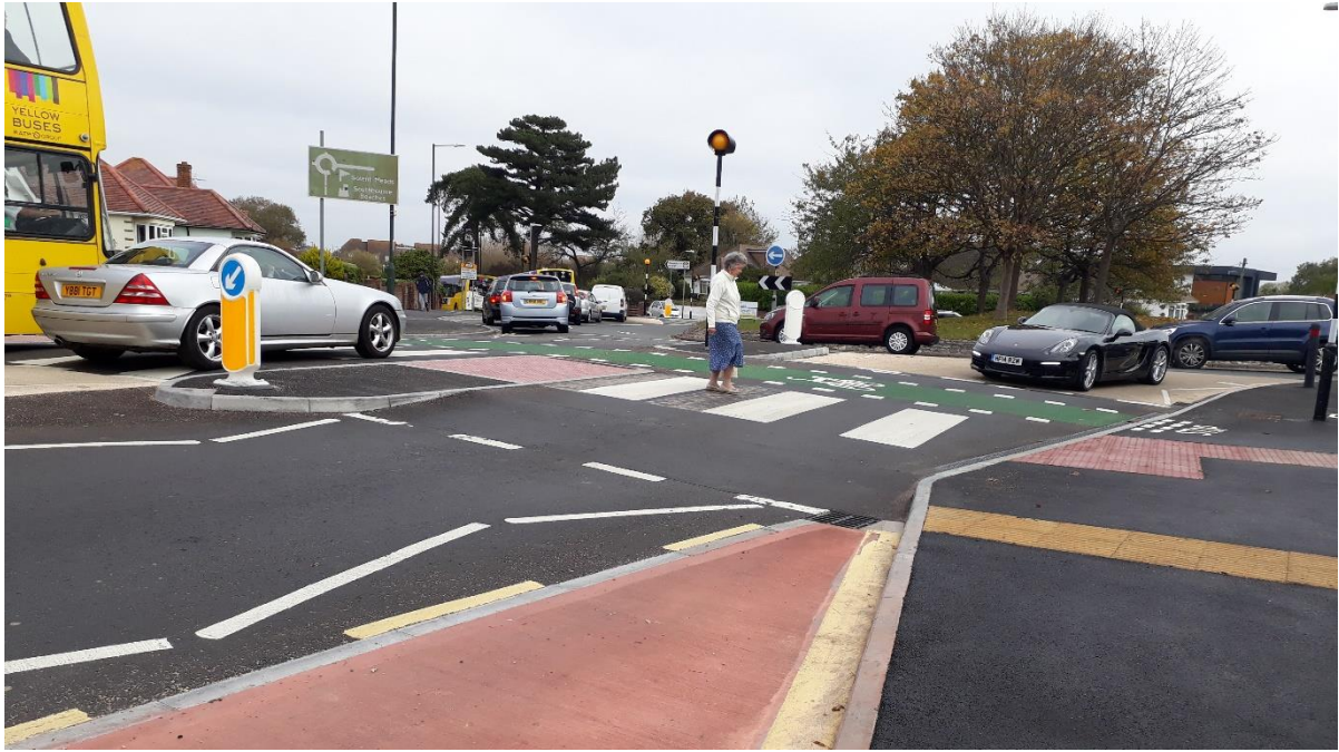
Figure 7: Prioritising pedestrians and cyclists. Parallel crossing on each arm of this roundabout to enable people to cross safely. Road safety scheme. Tuckton Roundabout, Bournemouth
