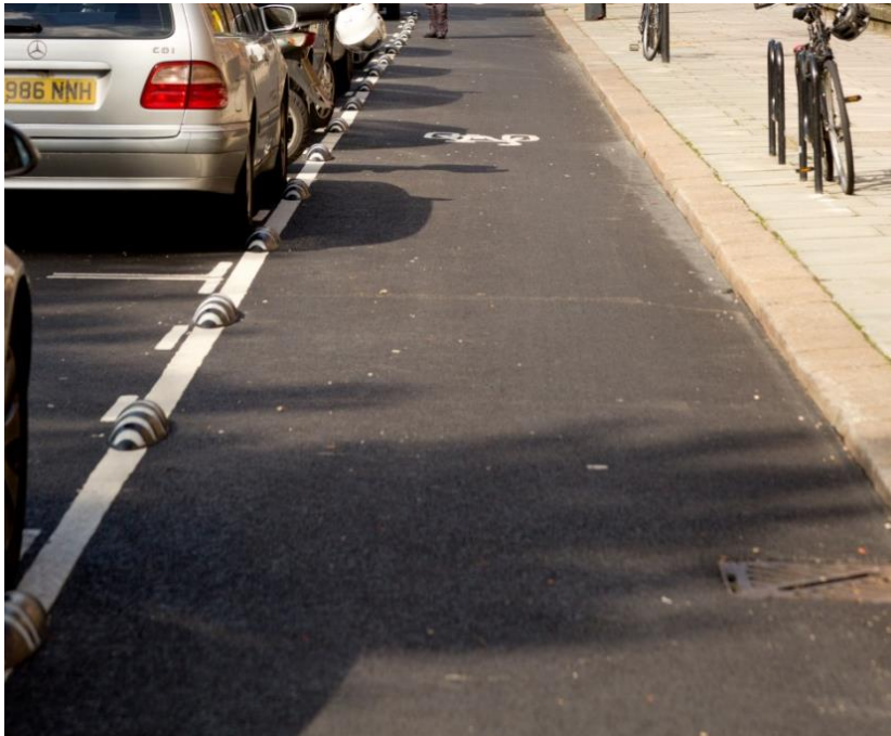
Figure 17: Light segregation or simply pushing out the parking is a cheap effective way to protect people cycling
