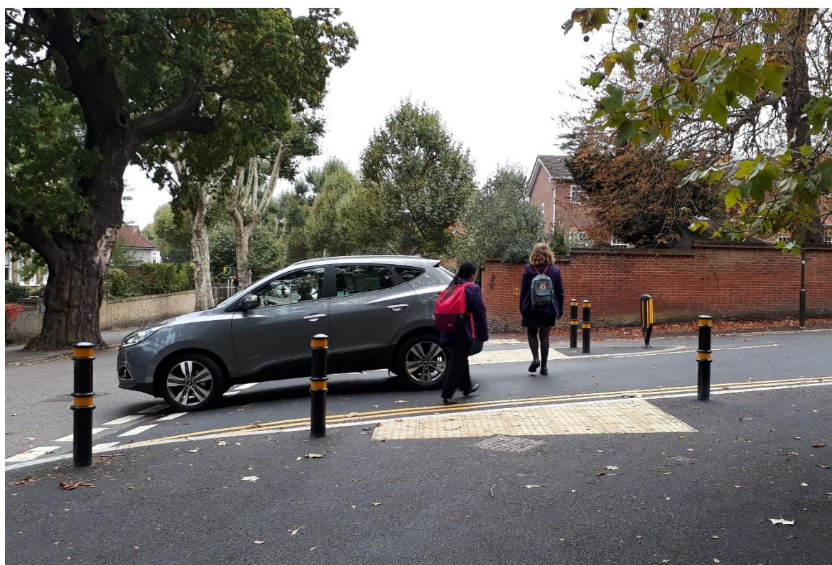
Figure 11: Newly configured side road junction, Lake Rd, Wimbledon. Driver assumes priority on turning into the newly reconfigured junction – a “safe route” school children? Kerb line follows path of motorist to ensure visual priority for driver not the pedestrian (in contravention with Highway Code Rule 170)
