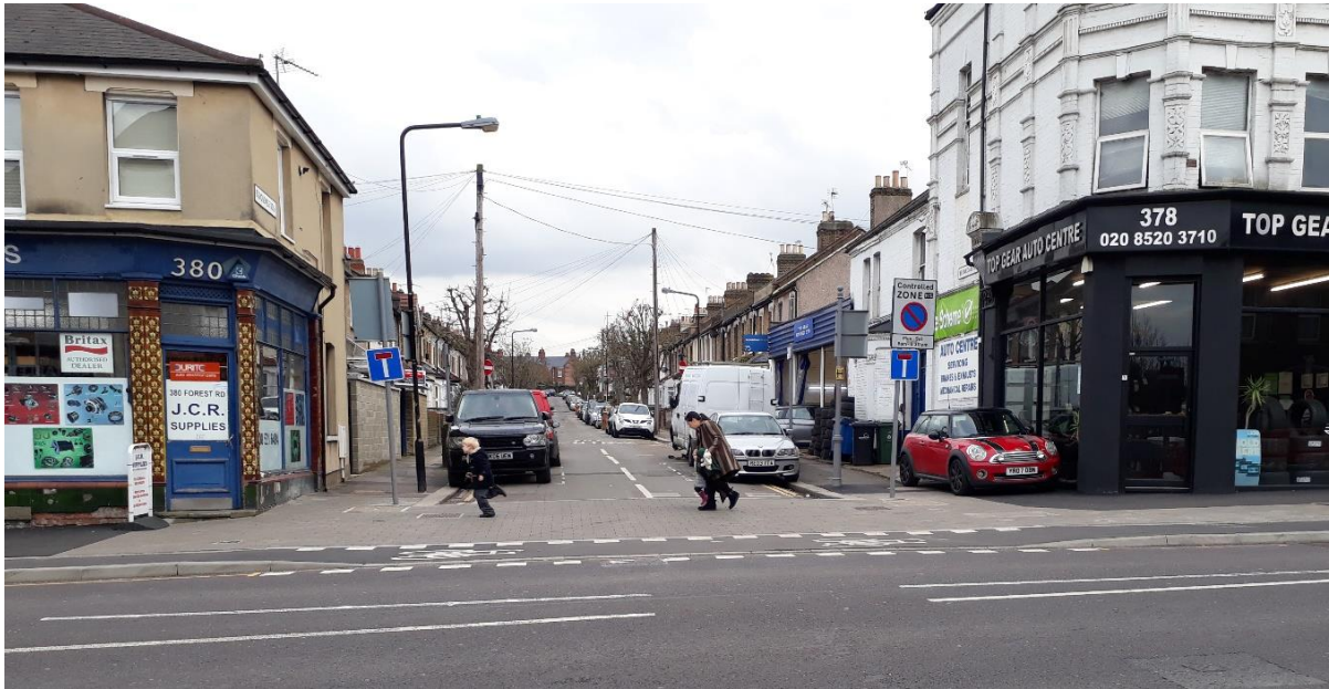
Figure 13: Recent design, Walthamstow, London: The kerb line follows the path of the pedestrian to provide visual priority to pedestrians (in line with Highway Code Rule 170) and reduced vehicle turning speeds so also assisting people cycling as well as walking.
