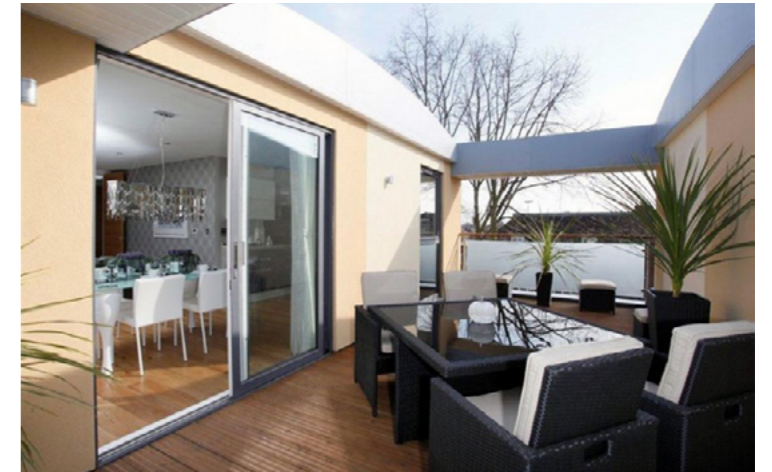
Fig.9.49 - Full height glazed doors leading on to balconies, which will minimise the need for artificial lighting. [Credit: Paul Murphy Architects]
