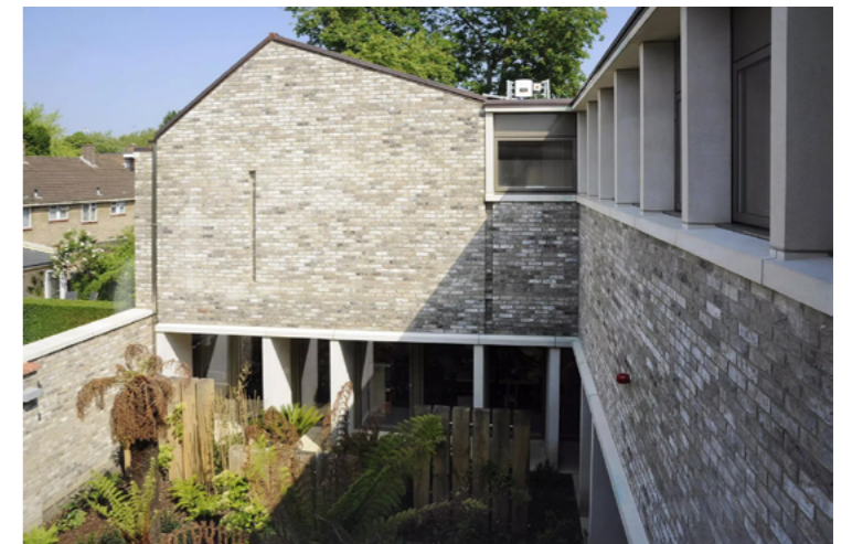
Fig.9.75 - Residents' access overlooking courtyard in the GP Surgery. [Credit: Panter Hudspith]
