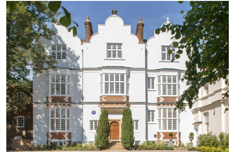
Fig.5.2 - A sensitive conversion and extension of a listed building to provide new homes. (Eagle House by Michaelis Boyd Associates ) [Credit: Octagon Developments]
