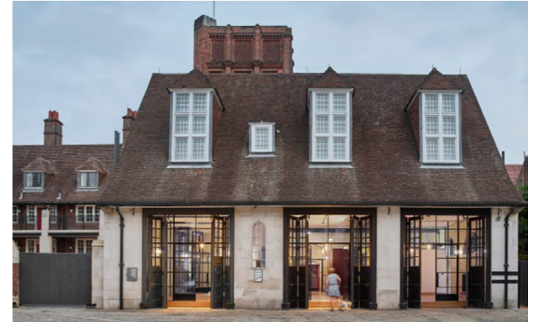
Fig.9.43 - Former engine bays converted into living space. [Credit: Kilian O'Sullivan]
