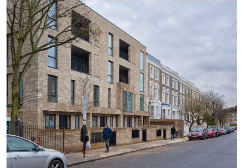
Fig.6.21 - A mix of home types in a compact building, it provides duplex's at street level with flats above. (Vaudeville Court, Islington by Levitt Bernstein ) [Credit: Tim Crocker]
