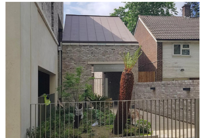
Fig.9.76 - Entrance to GP surgery is marked out by a form in keeping with neighbouring properties. [Credit: Panter Hudspith]
