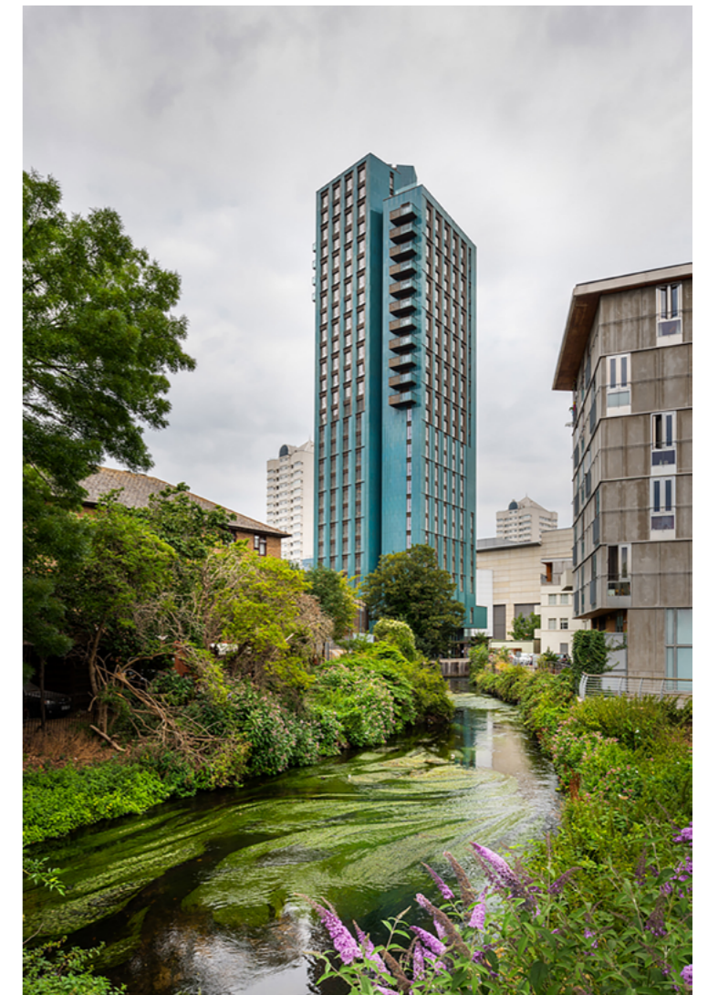
Fig.9.93 - View to tower from the river Wandle. [Credit: Simon Kennedy]
