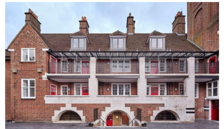
Fig.9.45 - Sensitive restoration of existing Grade II* fabric. [Credit: Kilian O'Sullivan]
