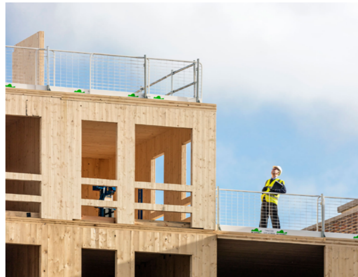
Fig.8.38 - This ground-breaking use of cross-laminated timber technology significantly reduced the carbon footprint of the building in terms of the amount of material used and energy consumption. (Dalston Works by Waugh Thistleton Architects ) [Credit: Waugh Thistleton Architects]
