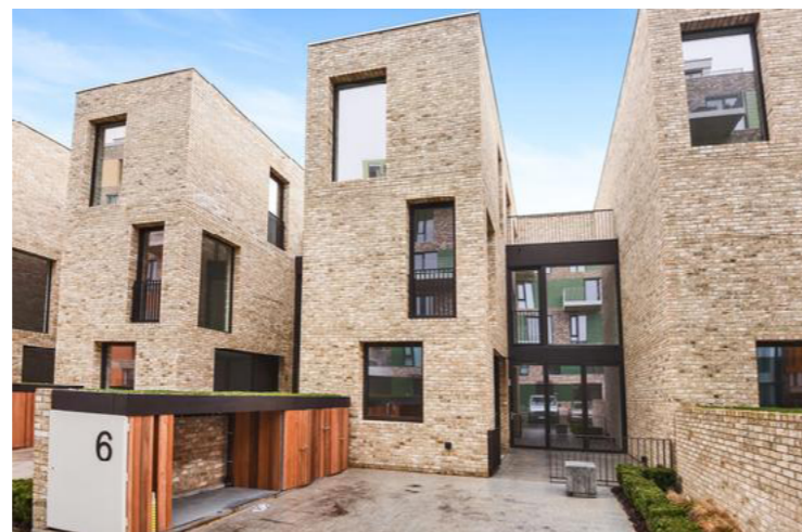
Fig.5.13 - Integrated bin and bike store. Storage for bins and bikes have been integrated into the landscape design of the front gardens. (Signal Townhouses, Greenwich by AHMM)
