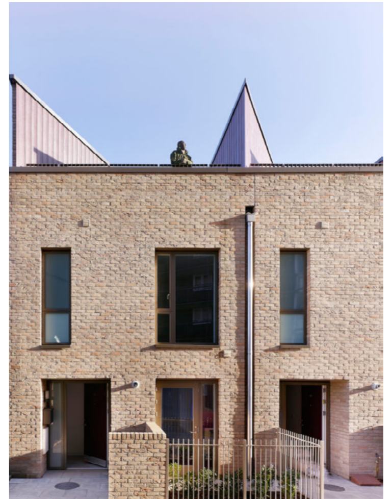
Fig.9.71 - View of front elevation and defensible space. [Credit: Bell Phillips Architecture]
