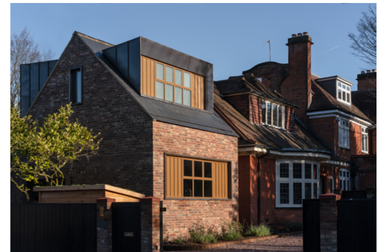
Fig.5.3 - A well detailed addition to a cottage built in 1906. (Dainton Cottage, Surbiton by WR-AP Architects )
