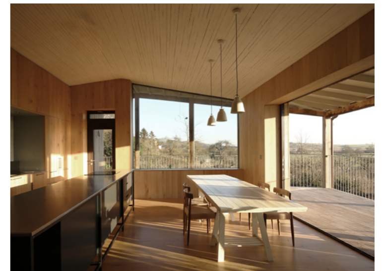
Fig.8.40 - Overhanging roof works in harmony with the energy strategy of this passivhaus by providing summer shading to the large areas of glazing positioned to the south-east. (Dundon Passivhaus by Prewett Bizley Architects ) [Credit: Passivhaus Trust / Prewett Bizley Architects]
