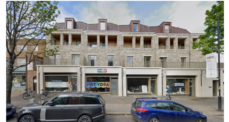
Fig.9.74 - Ground floor retail units continue the parade of shop fronts. [Credit: Panter Hudspith]
