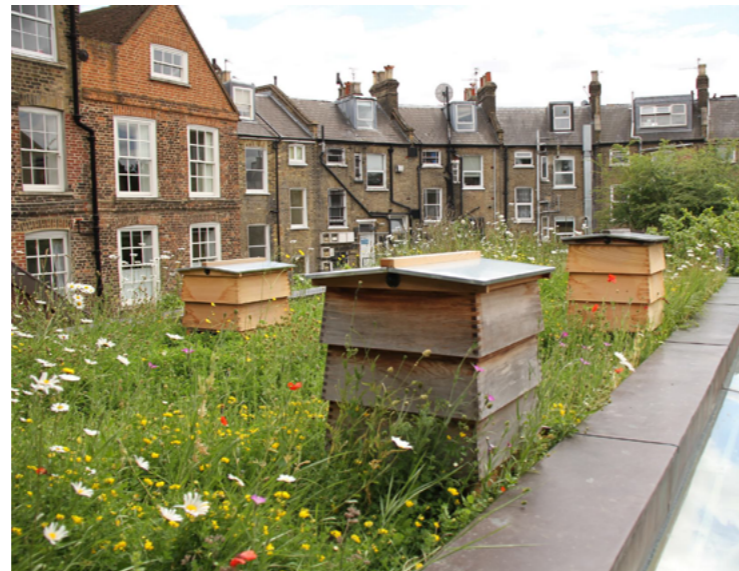
Fig.8.34 - The 4 green roofs of this backland home provides a diverse habitat for many plant and insect species in an urban environment. (The Muse by Bere:Architects) [Credit: Bere:Architects]
