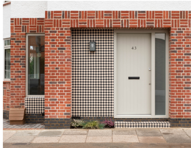
Fig.8.37 - New-build house references the terracotta brickwork as well as the Victorian tiling to front entrances of the neighbouring terrace homes. (Lucien road by Harp & Harp Architects ) [Credit: Harp & Harp Architects]
