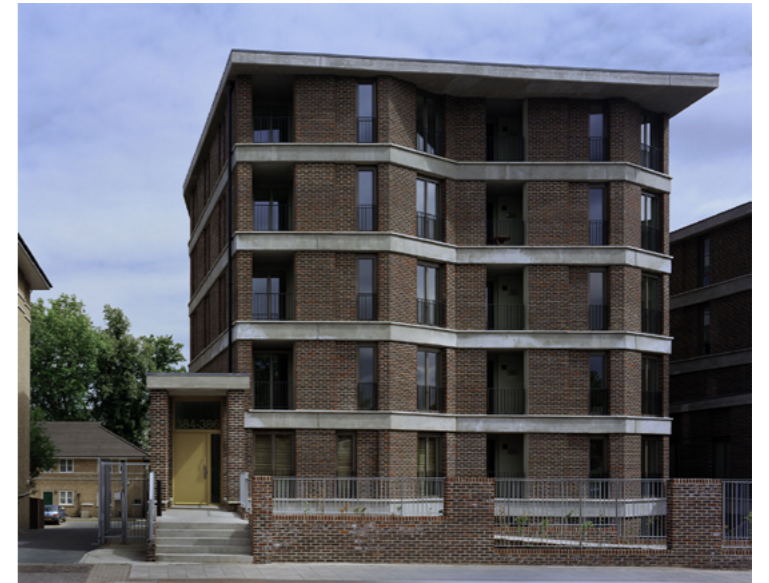
Fig.5.10 - The entrance of these villa blocks protrude towards the street and stand higher than the concrete banding marking each level. This creates a welcoming entrance that is distinct from other openings in the building fabric. (Finsbury Park Villas, Haringey by Sergison Bates Architects) [Credit: Stefan Müller]
