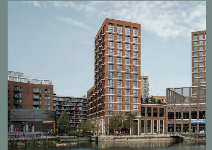
Porters Edge, Southwark © Maccreanor Lavington
