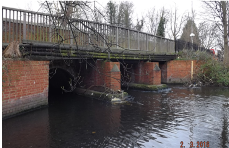
8. Upstream side: Bishopsford Road bridge, 2016, view looking north
