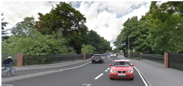
20. view of new bridge looking north (towards Mitcham town centre).
