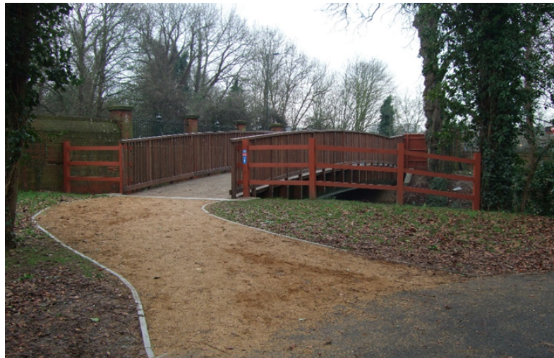
9. Downstream side, c2010, view looking north
