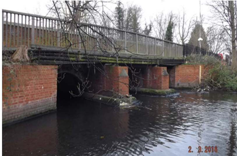
12. Upstream side: Bishopsford Road bridge, 2016, view looking north
