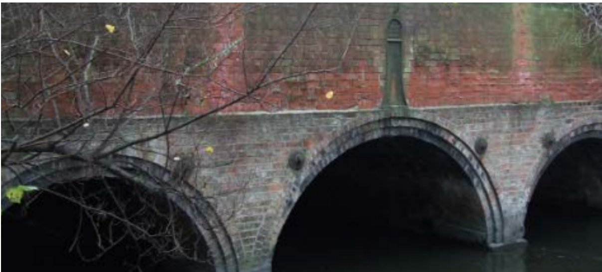
8. Mitcham Parish boundary marker on the west facing bridge parapet.
