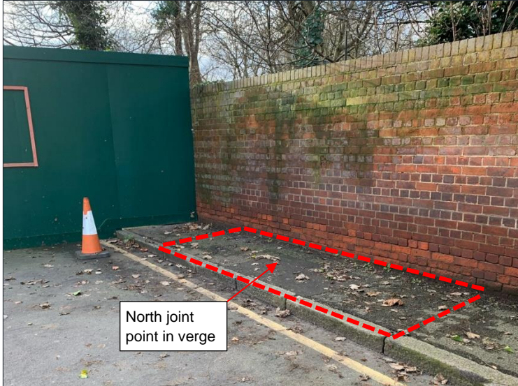
Figure 20 - Bishopford Road: anticipate location for commencement of HV / LV diversion
