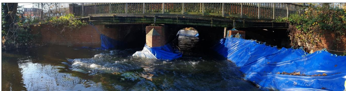
Figure 11 -East elevation showing temporary dam provision
