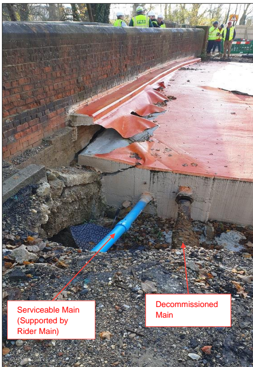
Figure 16 -Thames Water services adjacent to east parapet of arch bridge
