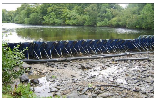
Figure 41 - Portadam details: as-constructed (l), erection and construction (r)
