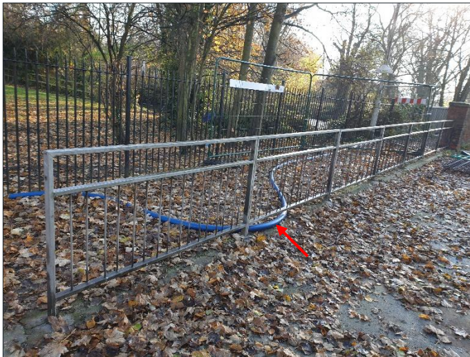
Figure 18 -Thames Water rider main – used to safeguard supplies through site [Left - Main at north east wingwall, Right: Across east (upstream) footbridge]
