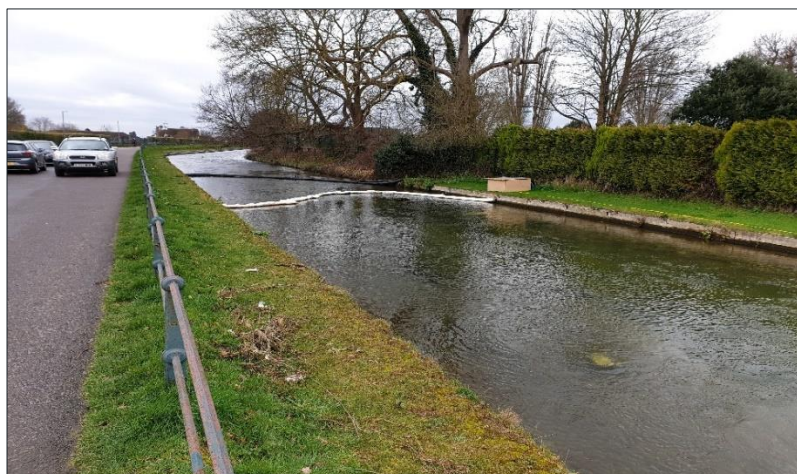
Figure 43 - Example in channel silt trap and oil boom
