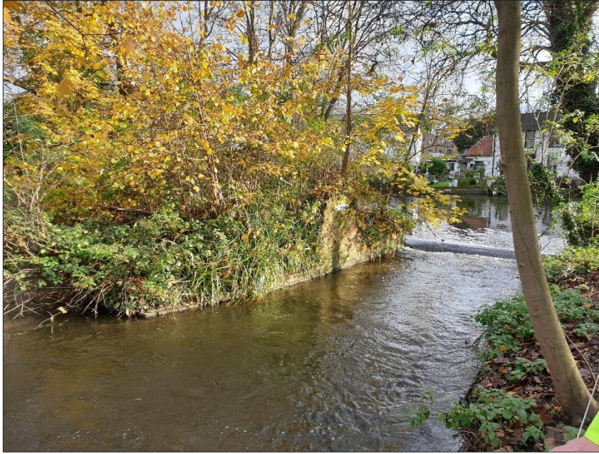
Figure 9 - View of weir upstream of Bishopsford Road Bridge
