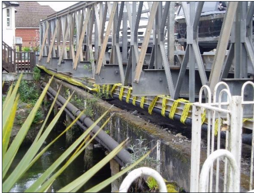
Figure 47 - Service routes supported from temporary bridge
