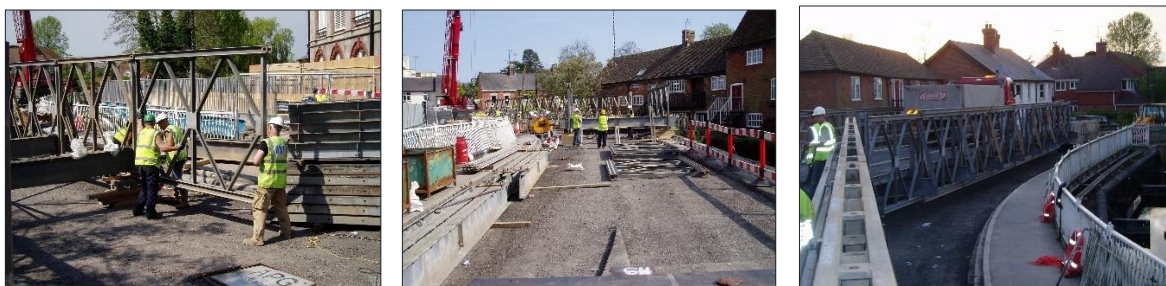
Figure 45 - Modular Bailey Bridge construction above existing bridge deck
