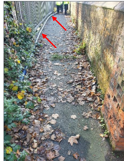
Figure 18 -Thames Water rider main – used to safeguard supplies through site [Left - Main at north east wingwall, Right: Across east (upstream) footbridge]
