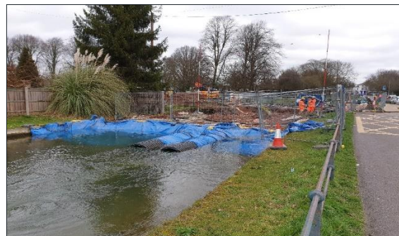
Figure 39 - Examples of dams formed in bagwork with through piping
