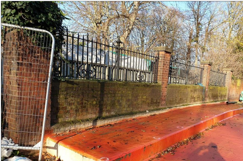
Figure 14 - West (downstream) elevation – inset parapet feature
