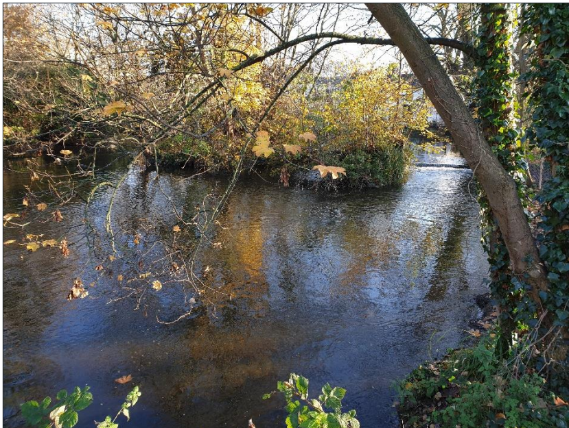
Figure 8 - View upstream along the River Wandle from south east wingwall
