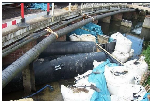
Figure 39 - Examples of dams formed in bagwork with through piping
