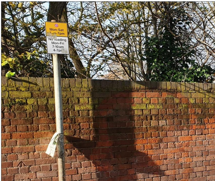
Figure 6 - Traffic restrictions on bridge approaches
